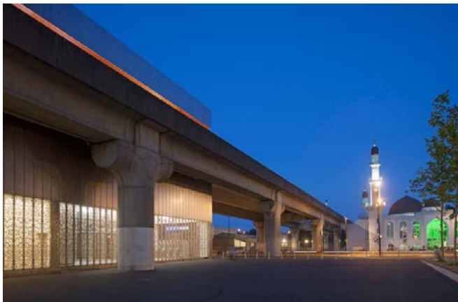
Station entrances (Kraaiennest Station, Amsterdam) Key station entrances provide important urban frontages, ensuring movement through the area has a positive civic dimension.
