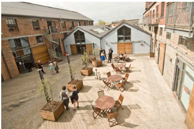
Mix (Paintworks, Bristol) A balanced mix of uses and scales offers the potential to activate the area, by intensifying the land use.
