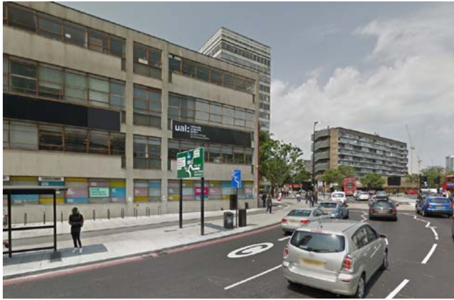
Improve carriageway width (Newington Butts, London) A rebalancing of the relationship between vehicles, cycles and pedestrians can improve connectivity.
