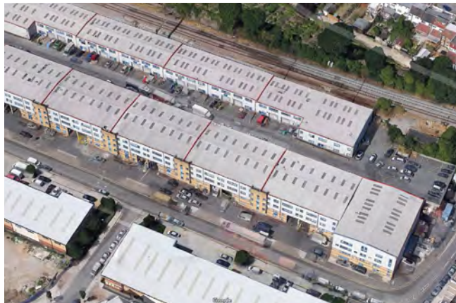
Multi-storey industry, Theydon Road, Hackney
