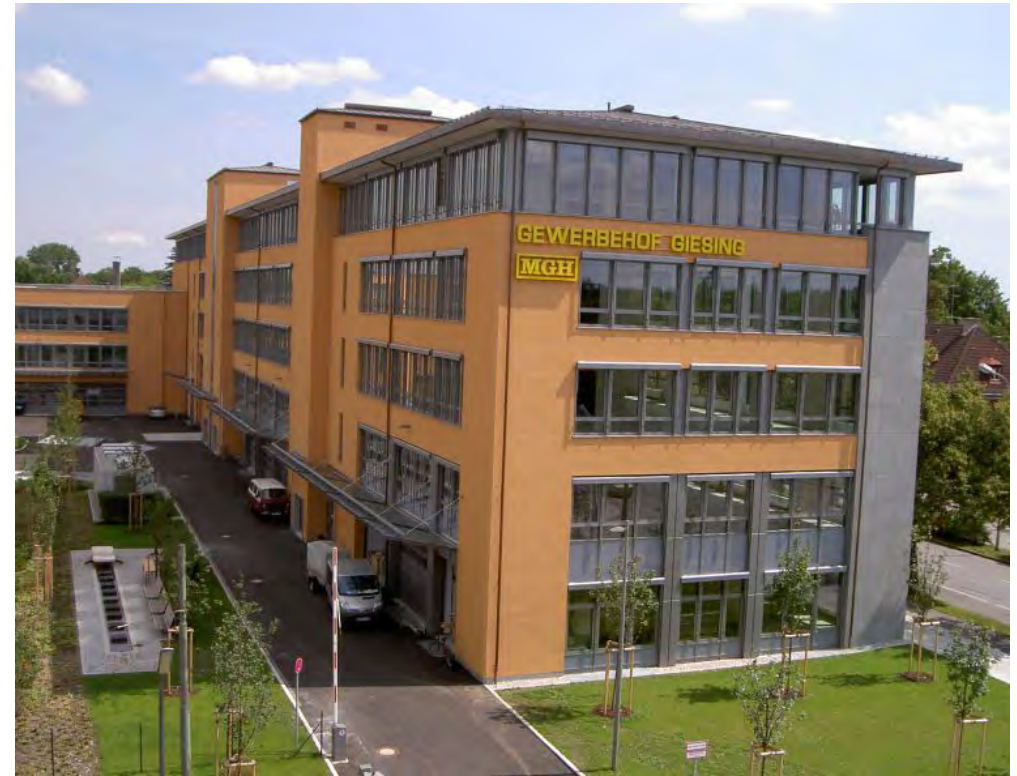
High density workspace, Munich
