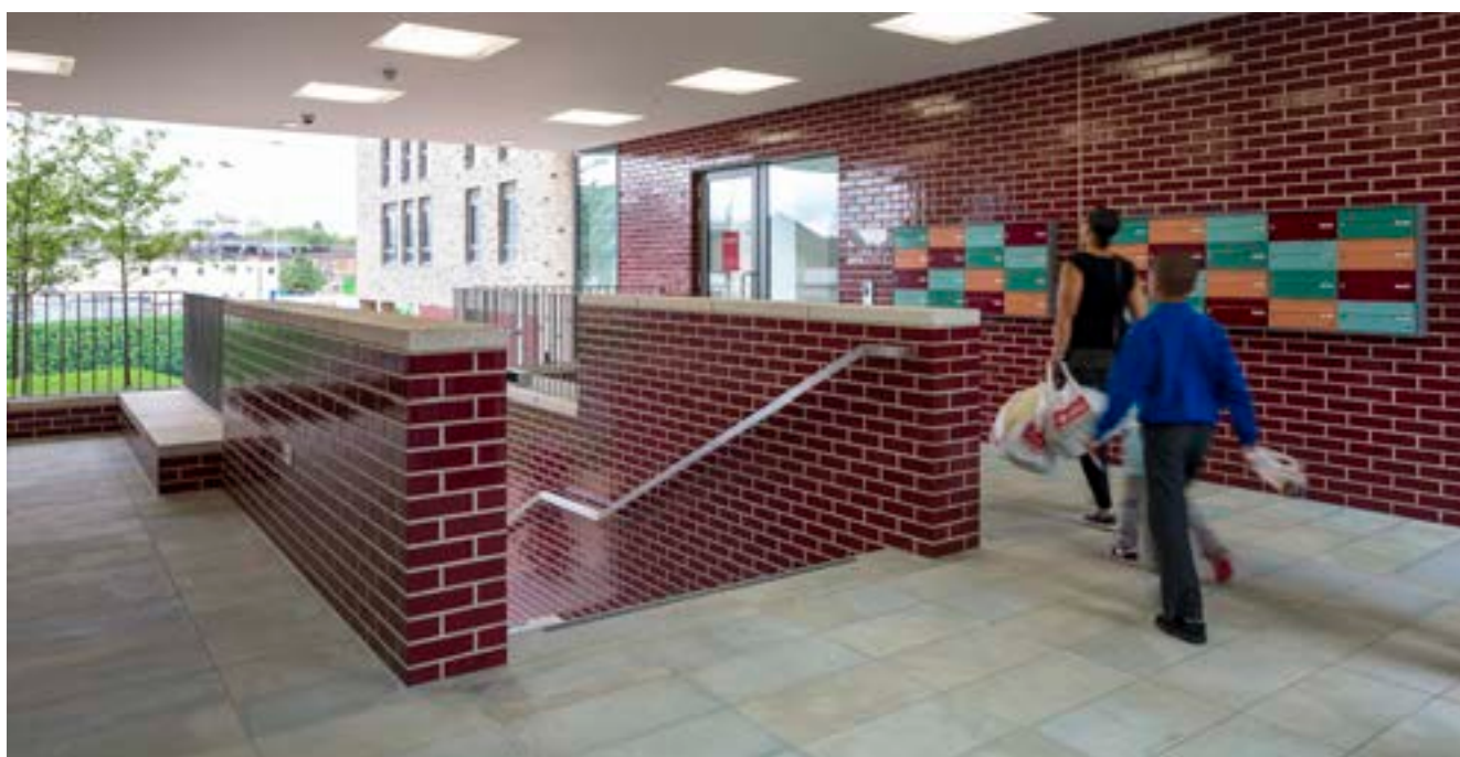
GROUND LEVEL SERVICING: RUBICON COURT, KING'S CROSS CENTRAL
