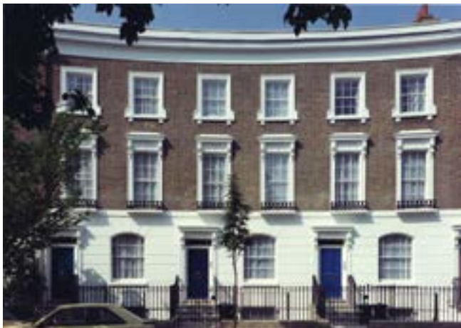
DENSITY: 1848 - 32 DPH / 1987 - 96 DPH THORNHILL SQUARE, ISLINGTON: BUILT 1848, RESTORED & CONVERTED 1987
