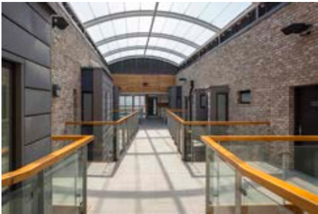
ATRIUM ACCESSED APARTMENTS: ROFFO COURT, AYLESBURY ESTATE
