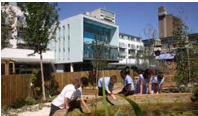
FLATS OVER A SCHOOL: ST THOMAS' CE PRIMARY SCHOOL, KENSINGTON
