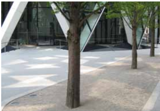
Well-maintained loose gravel provides porous surround for trees at 30 St Mary Axe, London. Image: Capita
