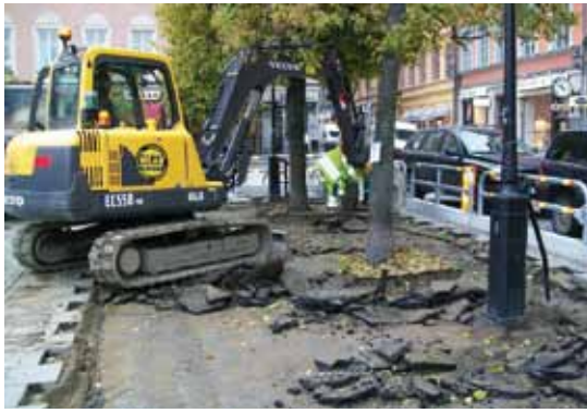
Excavations start on Kornhamnstorg a public square in Stockholm's old town where lime trees show early sign of decline.
