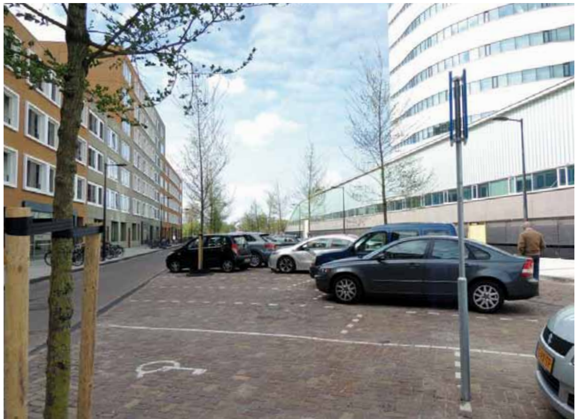
Newly installed permeable paving laid over a raft system (Permavoid Sandwich Construction) in Amsterdam, The Netherlands. Image: Jeremy Barrell
