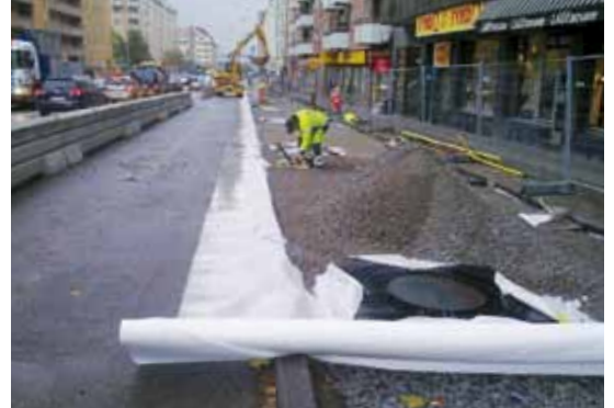
A geotextile separates the aeration layer (dry stones, smaller grade) placed above the skeleton stone-soil mix, and the paving sub-base.
