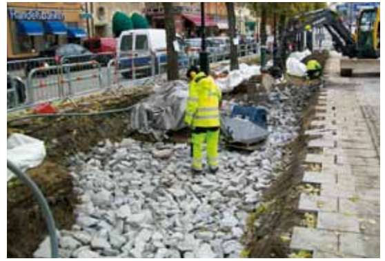
Large stones for the skeleton soil layer are being positioned and compacted in the newly created continuous trench.
