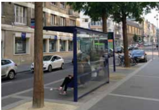
Porous self-binding aggregate surrounds trees near bus stop in Rouen, France.
