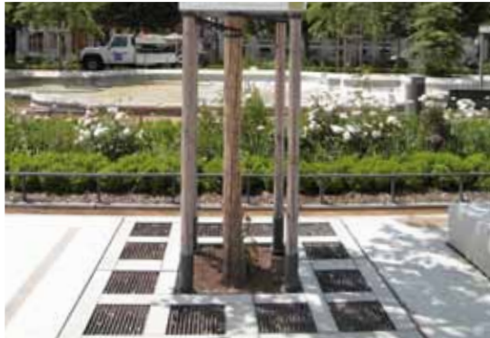
Tree grille with limestone infill at 90 degrees to pedestrian flow to reduce slipping, aids water infiltration and gas exchange. Place de Bellecour, Lyon, France.
