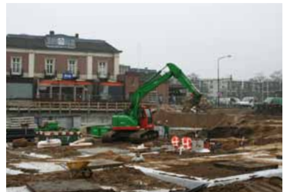
Protective covers are placed over planting holes.
