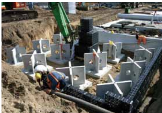
Placing cellular units around concrete crates.
