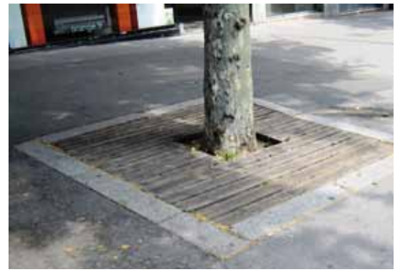
The opening of timber tree grates can easily be resized or tailored to accommodate trunk growth or mature trees. Lyon, France. Image: Frédéric Ségur
