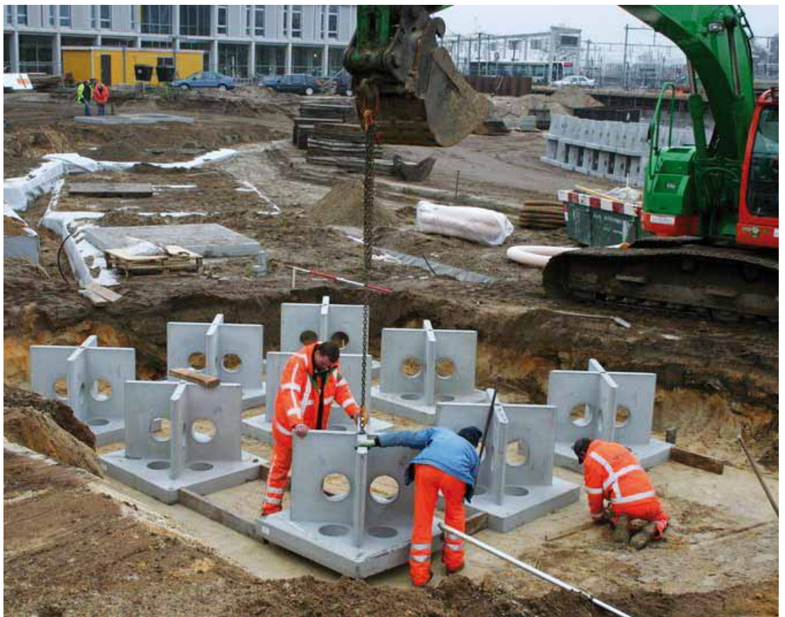
Positioning concrete crates on prepared island base at Apeldoorn station square (see Case study 24, p127).
