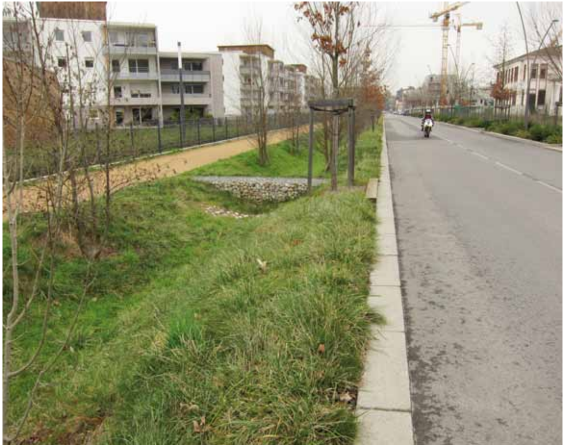
Swale between carriageway and footway in Sathonay near Lyon, France. Image: Richard Barnes
