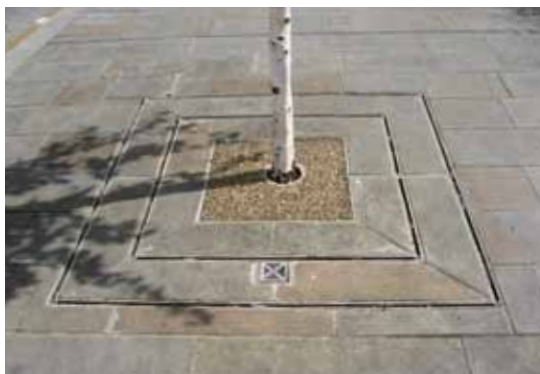
Grate with watering/aeration inlet and York stone infill matches surrounding paving at busy Dalston Junction bus station in Hackney, London.
