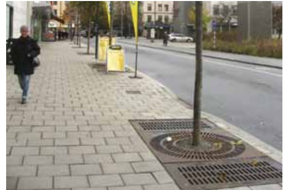
Extensive ductile cast iron grate facilitates water infiltration and effective gas exchange between above- and below-ground environments in Stockholm, Sweden.
