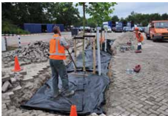
Trees planted, geotextile in place to prepare the foundation for the concrete block pavers.
