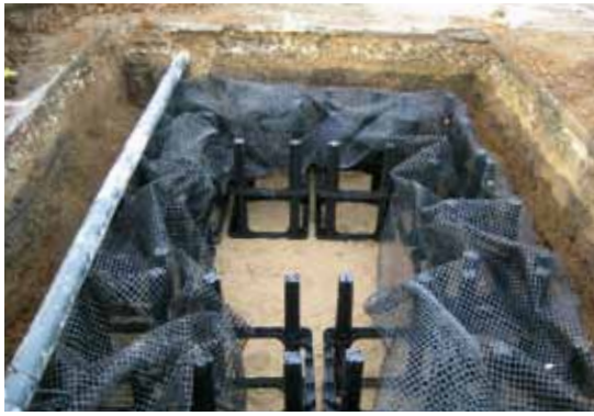
Placing the crates, accommodating the water main (see Case study 9, p38).
