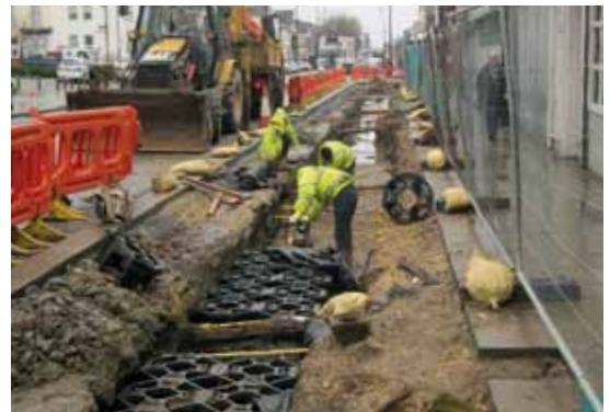
Compacting base and placing crates.
