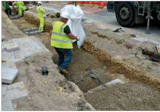
Drainage layer and root ball anchoring system.
