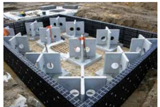
Island ready for soil fill.
