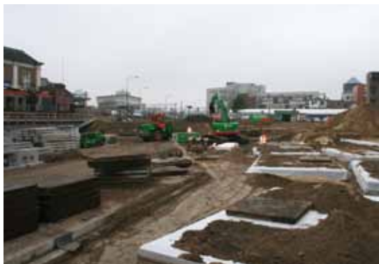
Filled islands topped with geotextile.
