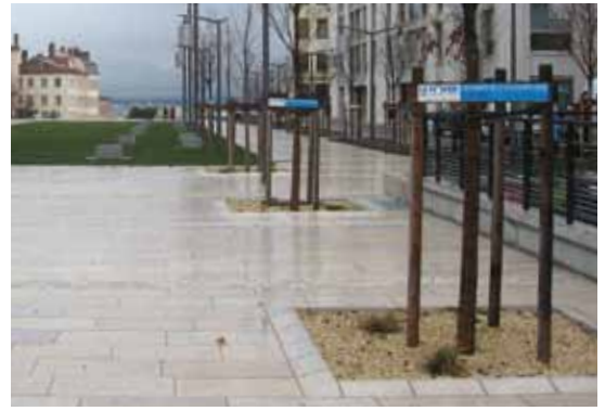
A gentle lip at the edge of the surface opening discourages trespassing and keeps wood shavings in place. Lyon, France.
