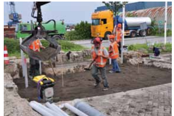
Filling with 100% recycled sand-based structural soil in 30 cm layers, well compacted with a vibrating (wacker) plate.
