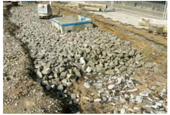
Soil has been flushed into the first layer of compacted large stones. A second layer of large stones is being applied.
