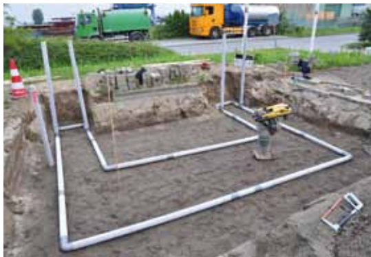
Site excavated and aeration system in place.
