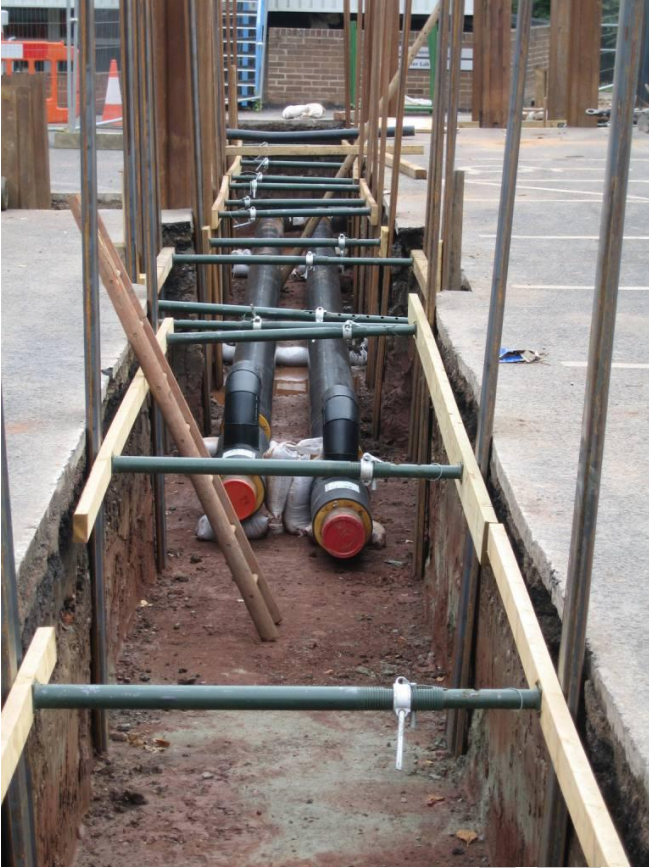
Figure 4.1 – Trench wall supports (reproduced courtesy of AECOM)
