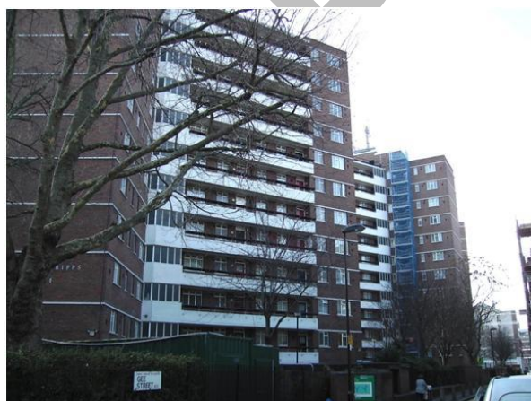
Figure 4 - Existing buildings supplied by a new Heat Network – Stafford Cripps Estate Islington
