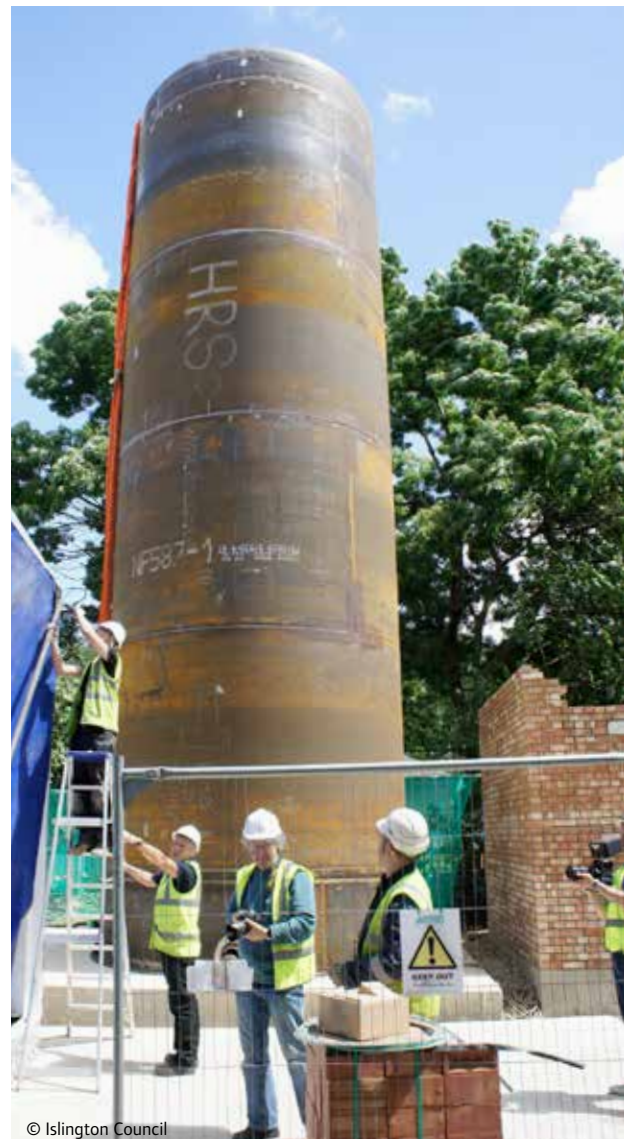
Figure 11. Thermal storage vessel during early phase of installation
