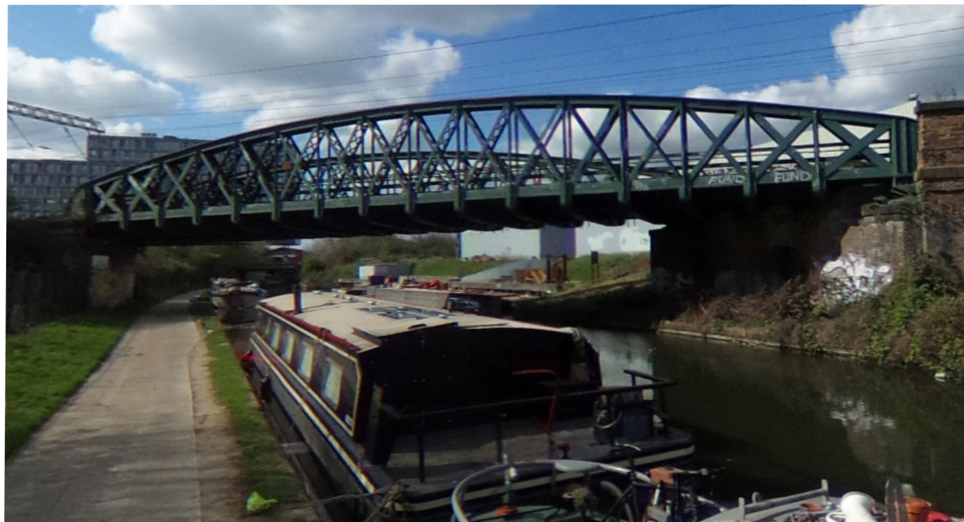
Figure 48: Existing bridge over a canal
