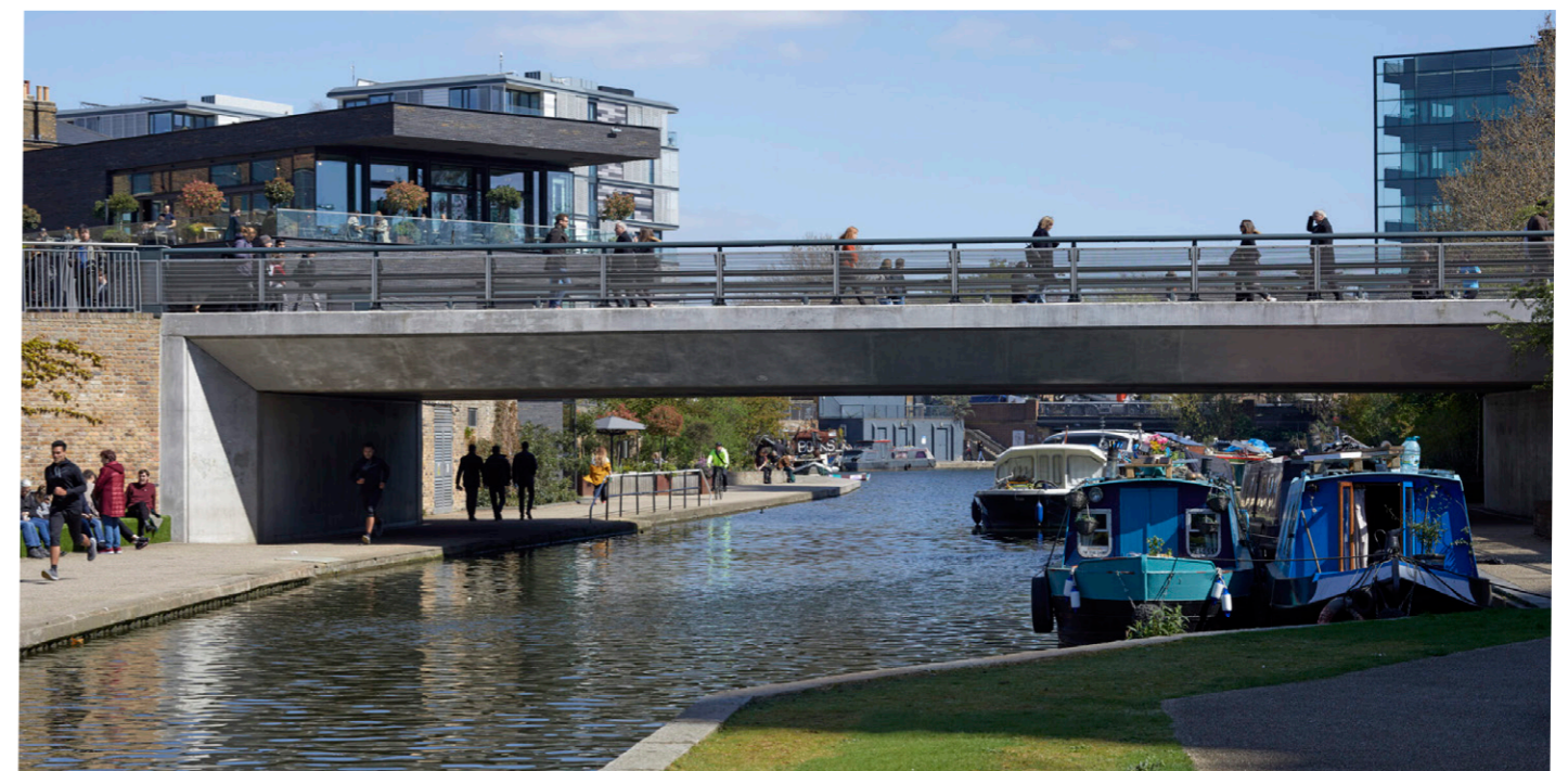
Figure 32: Regents Canal Bridge, a concrete bridge. Source: Knights Architects
