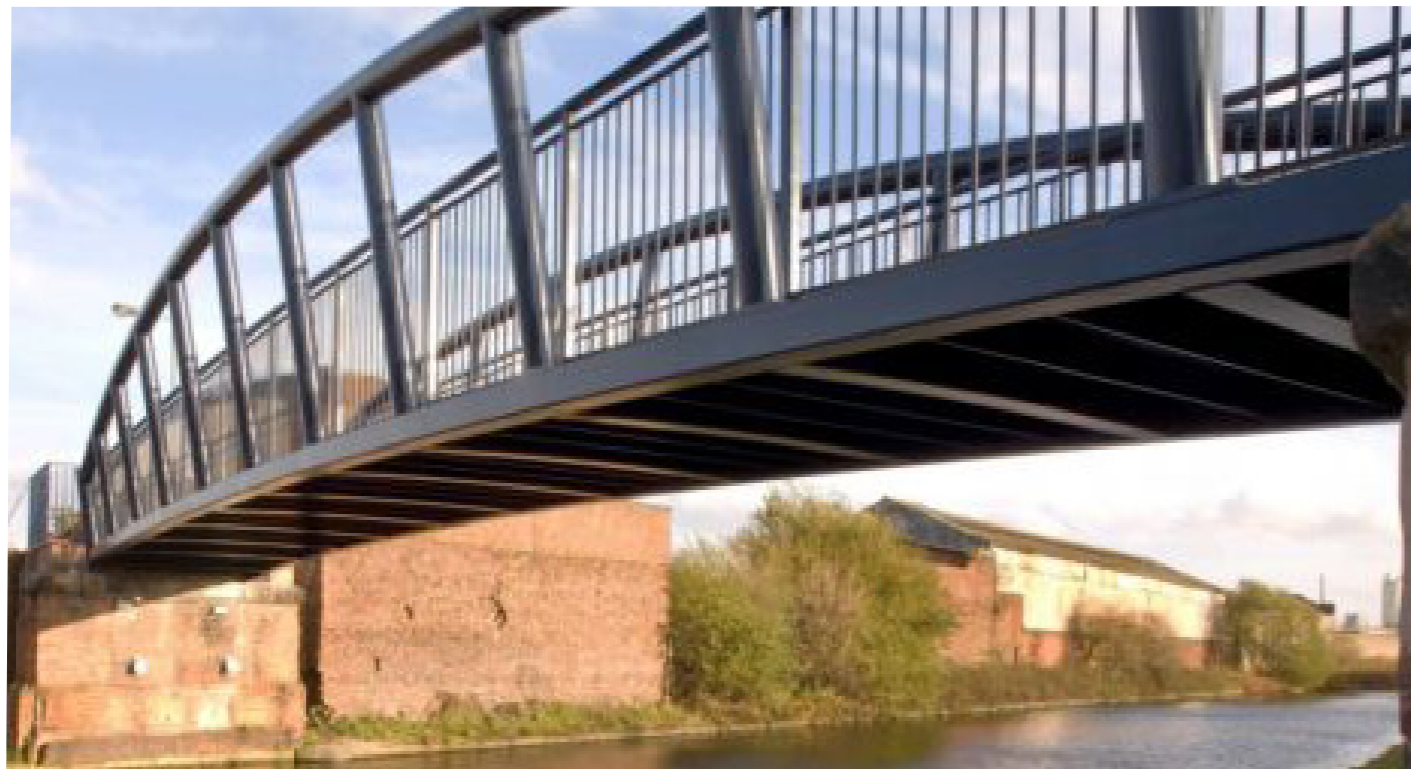
Figure 38: Bowstring bridge. Source: CTS Bridges Ltd.
