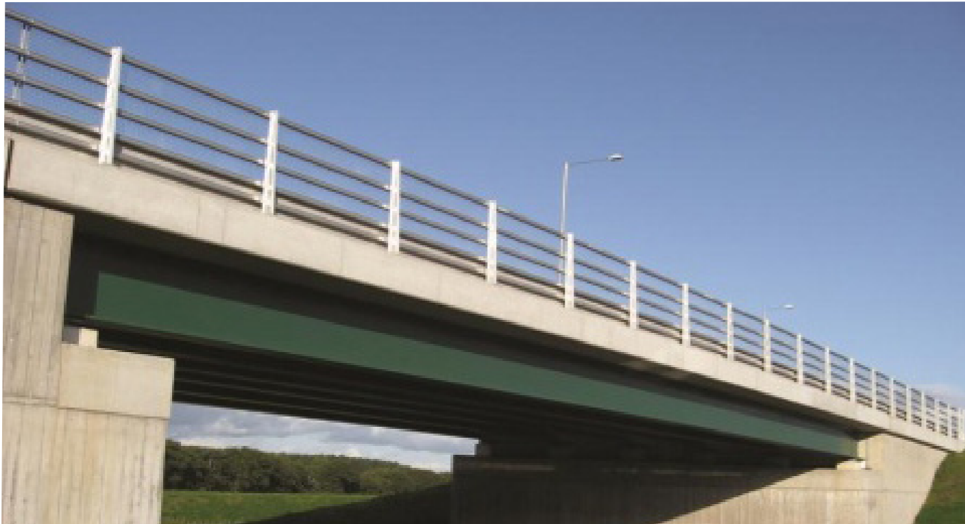
Figure 33: A typical multi beam bridge completed. Source: steelconstruction.org
