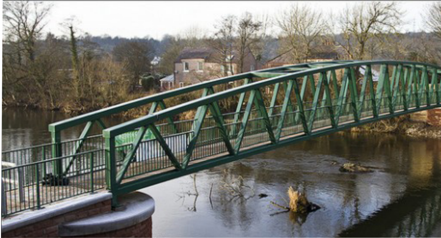
Figure 7: Camerton Footbridge. Source: NuSteel Structures Ltd.
