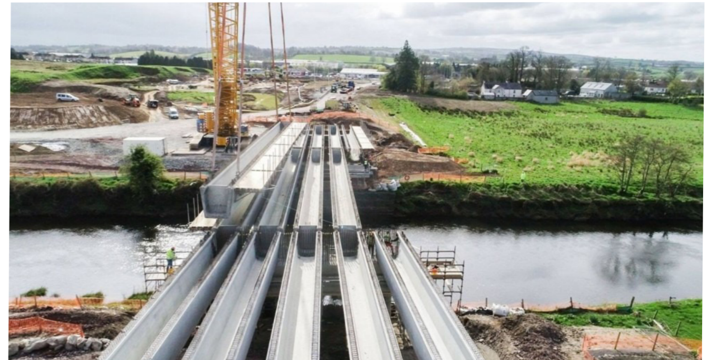
Figure 31: Concrete composite bridge using W type beams. Source: Shay Murtagh Ltd.
