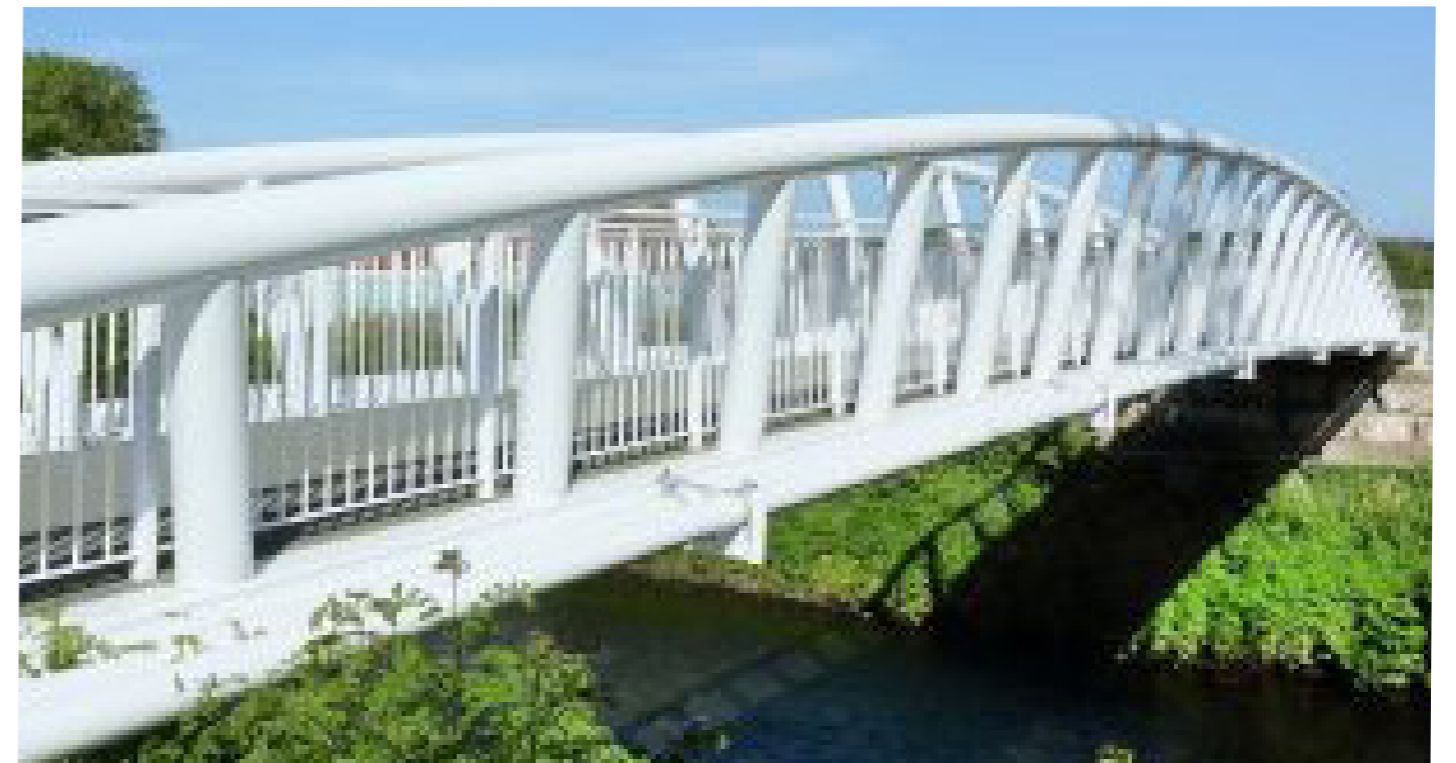
Figure 50: Example of a bridge structure over a canal Source: CTS Bridges Ltd
