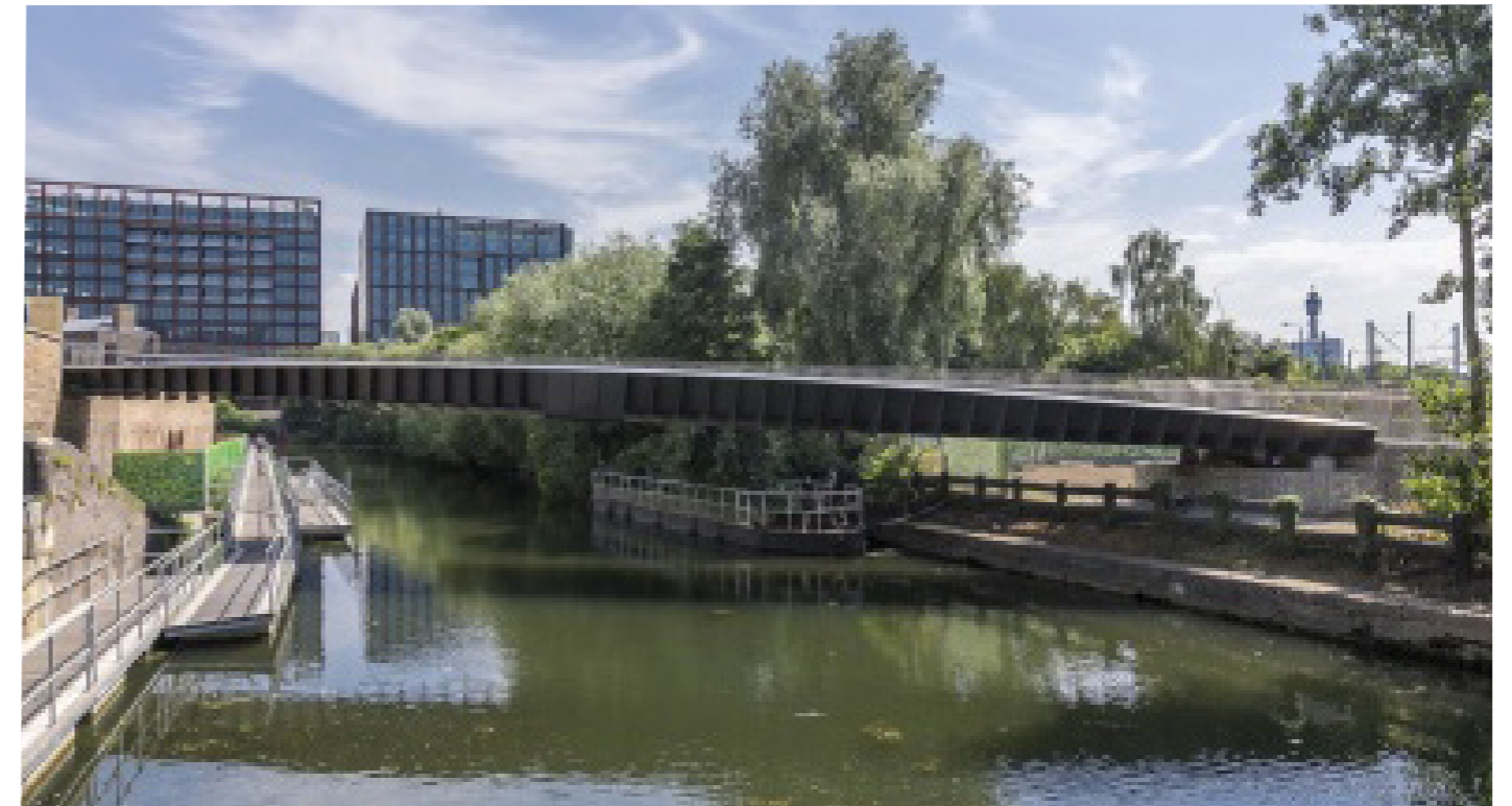
Figure 39: Somers Town Link Bridge, at King's Cross, spanning the Regents Canal, this is a "half-through" structure Source: steelconstruction.org
