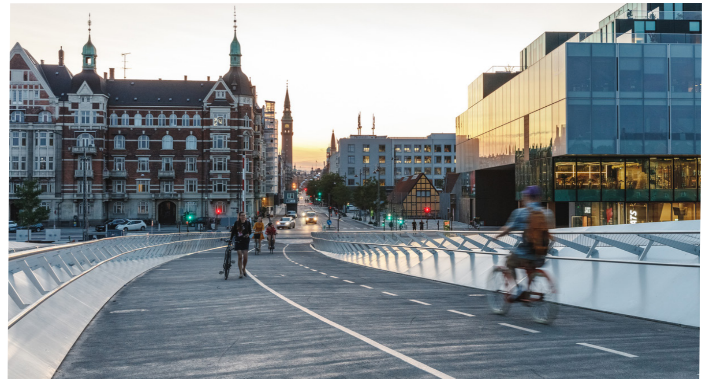
Figure 6: Lille Langebro cycle and pedestrian bridge; Copenhagen, Denmark
