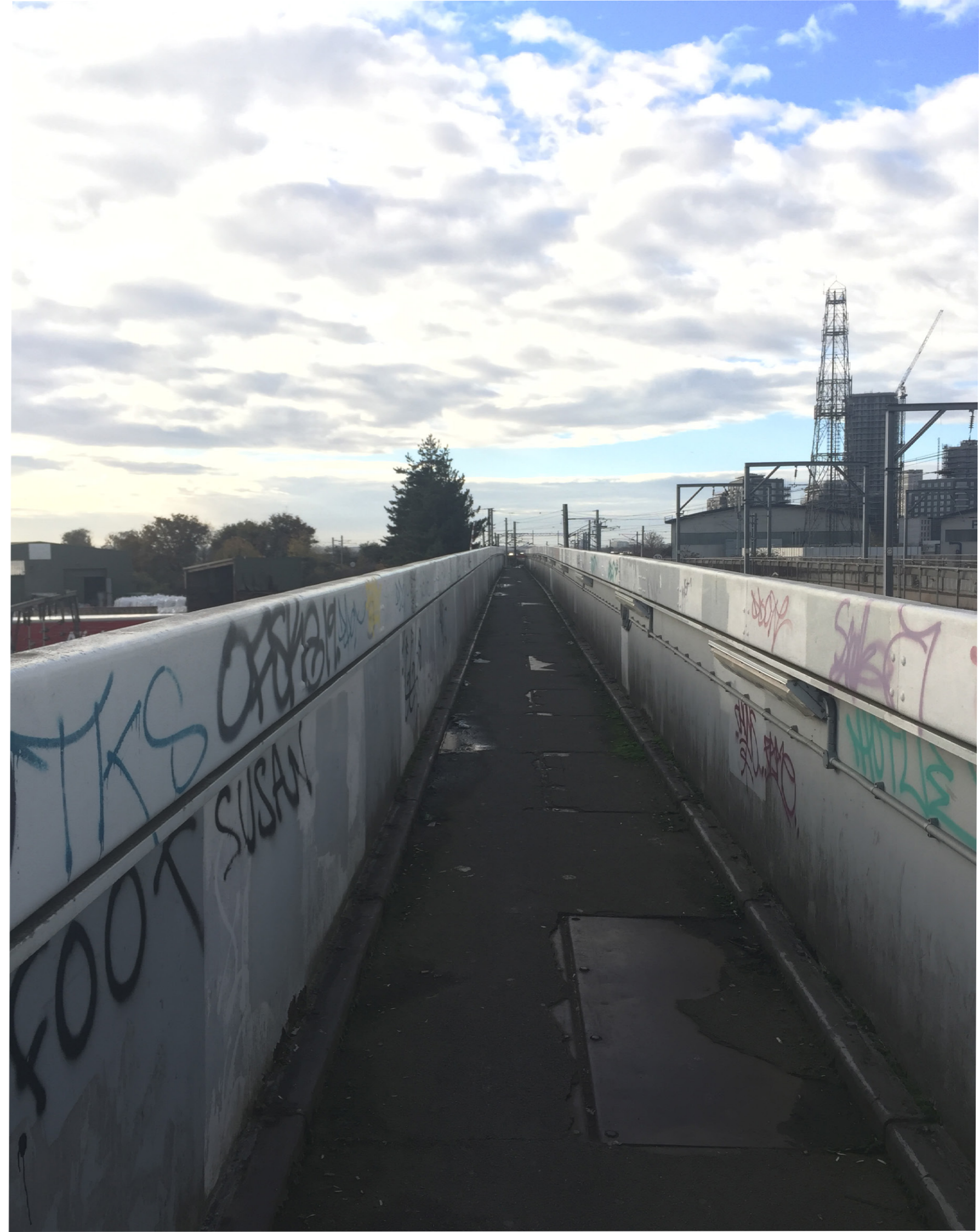
Figure 55: The current footbridge between Willesden Junction station and Old Oak North
