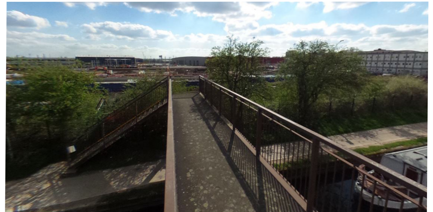
Figure 52: Existing pedestrian bridge over a canal
