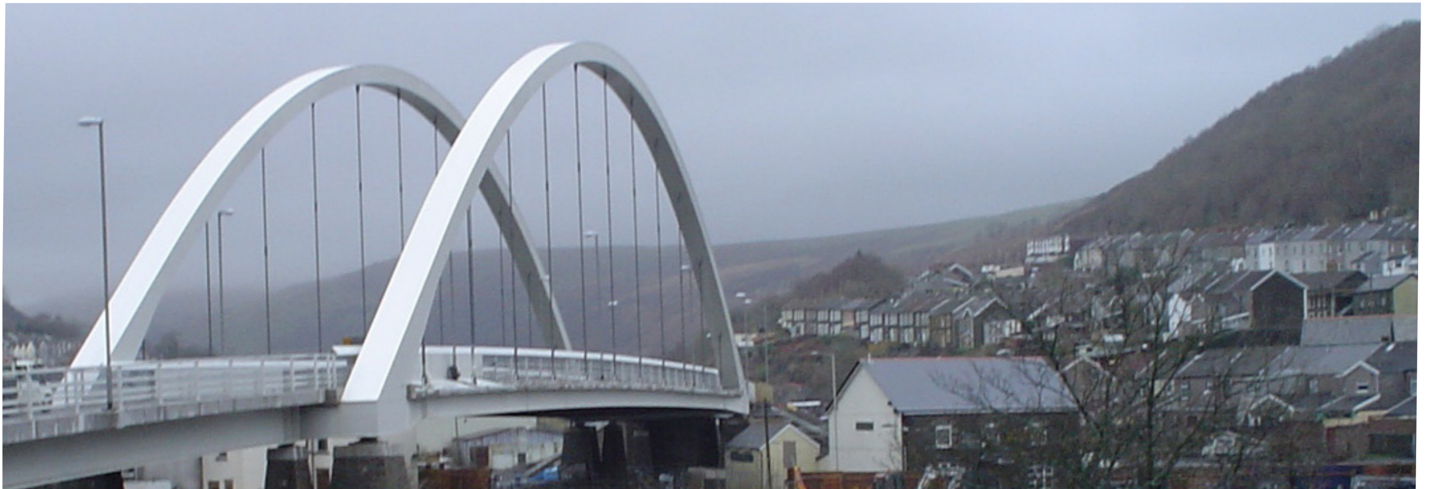
Figure 35: A “tied-arch” structure.
