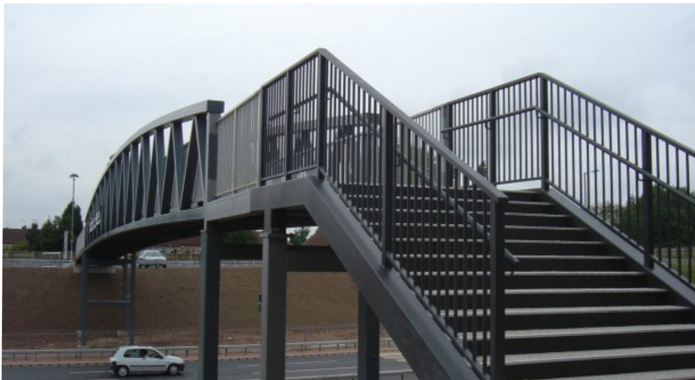
Figure 8: Phoenix Way Footbridge. Source: NuSteel Structures Ltd.
