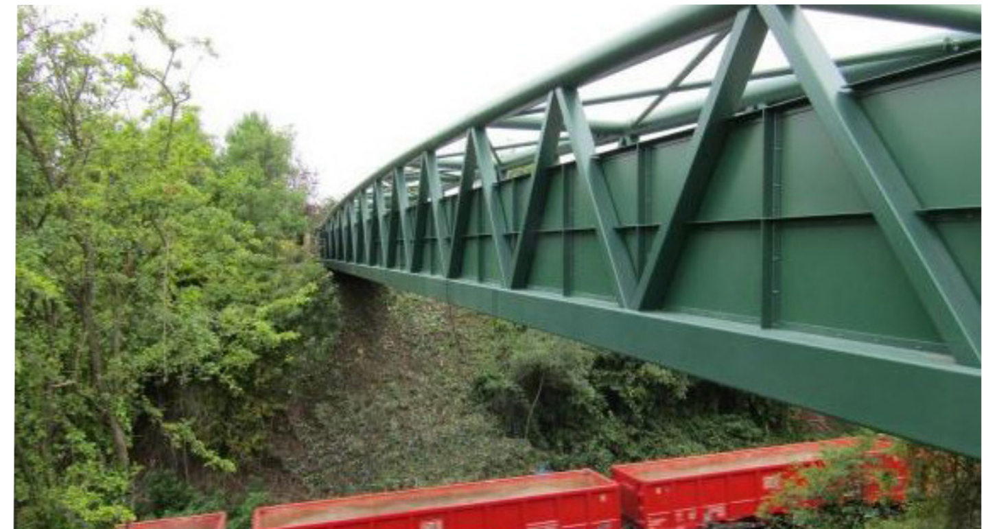
Figure 10: Warren Truss cycle bridge over a railway line. Source: CTS Bridges Ltd.
