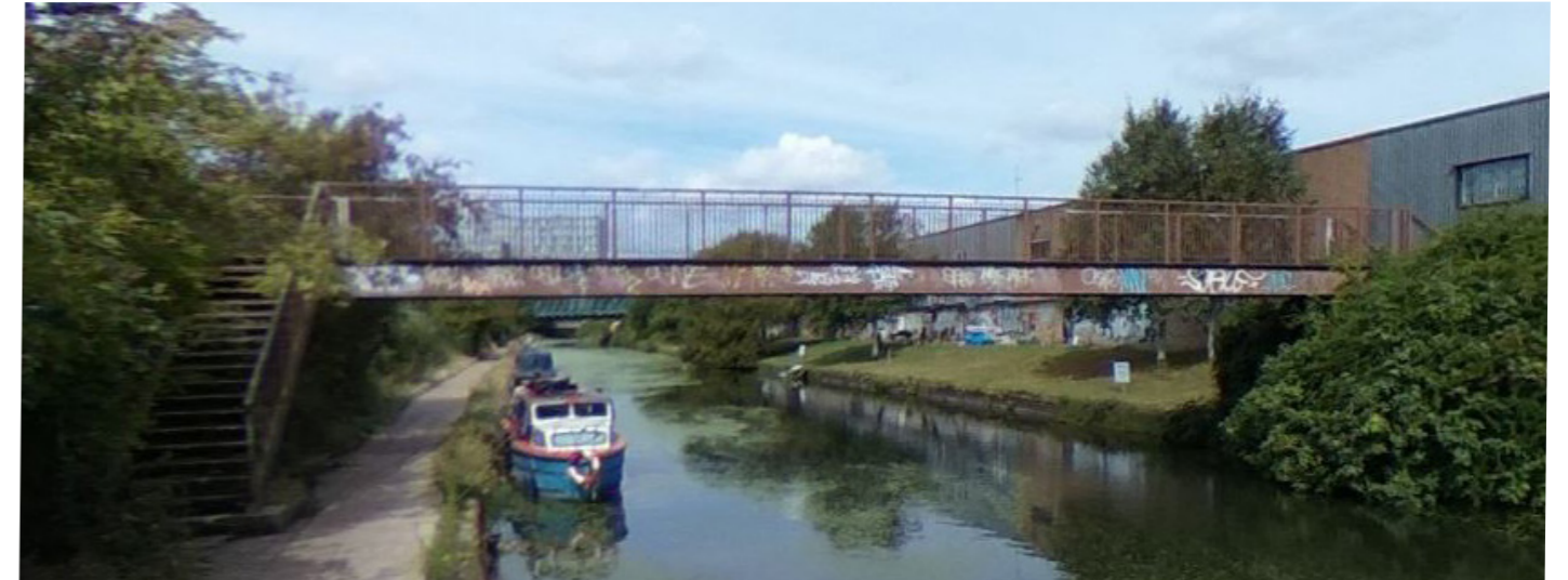
Figure 51: View of the existing pedestrian bridge over a canal
