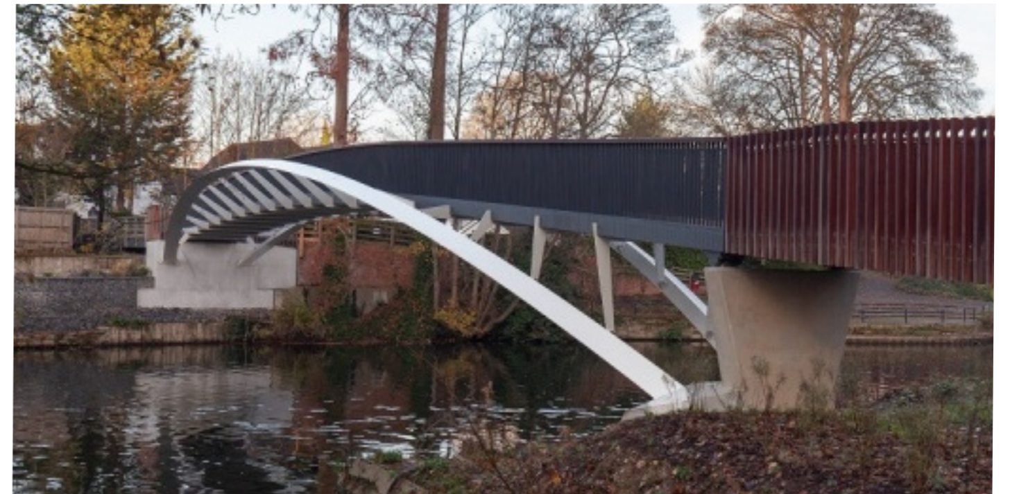
Figure 49: Existing bridge example Source: CTS Bridges Ltd
