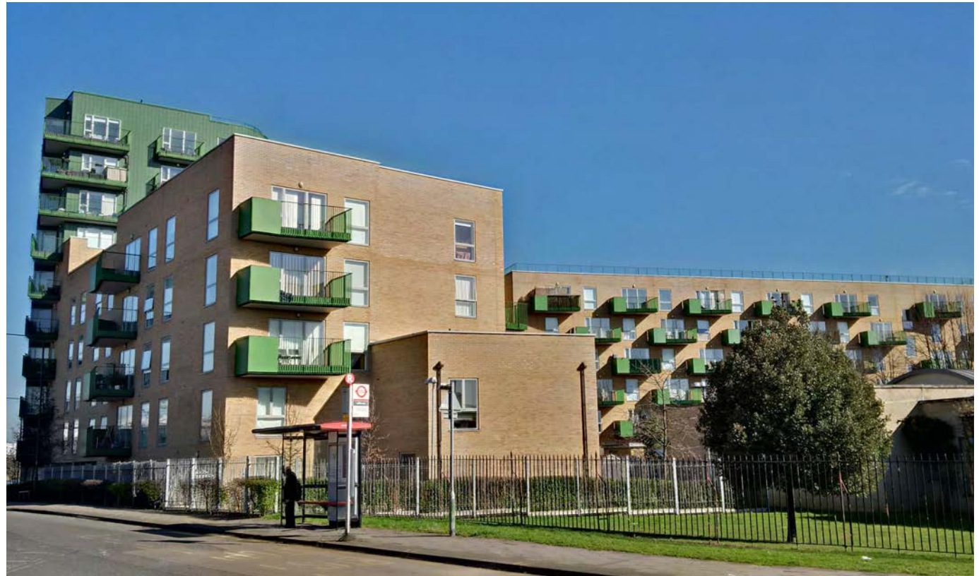
Figure 4.20: Recent residential development within Park Royal Centre
