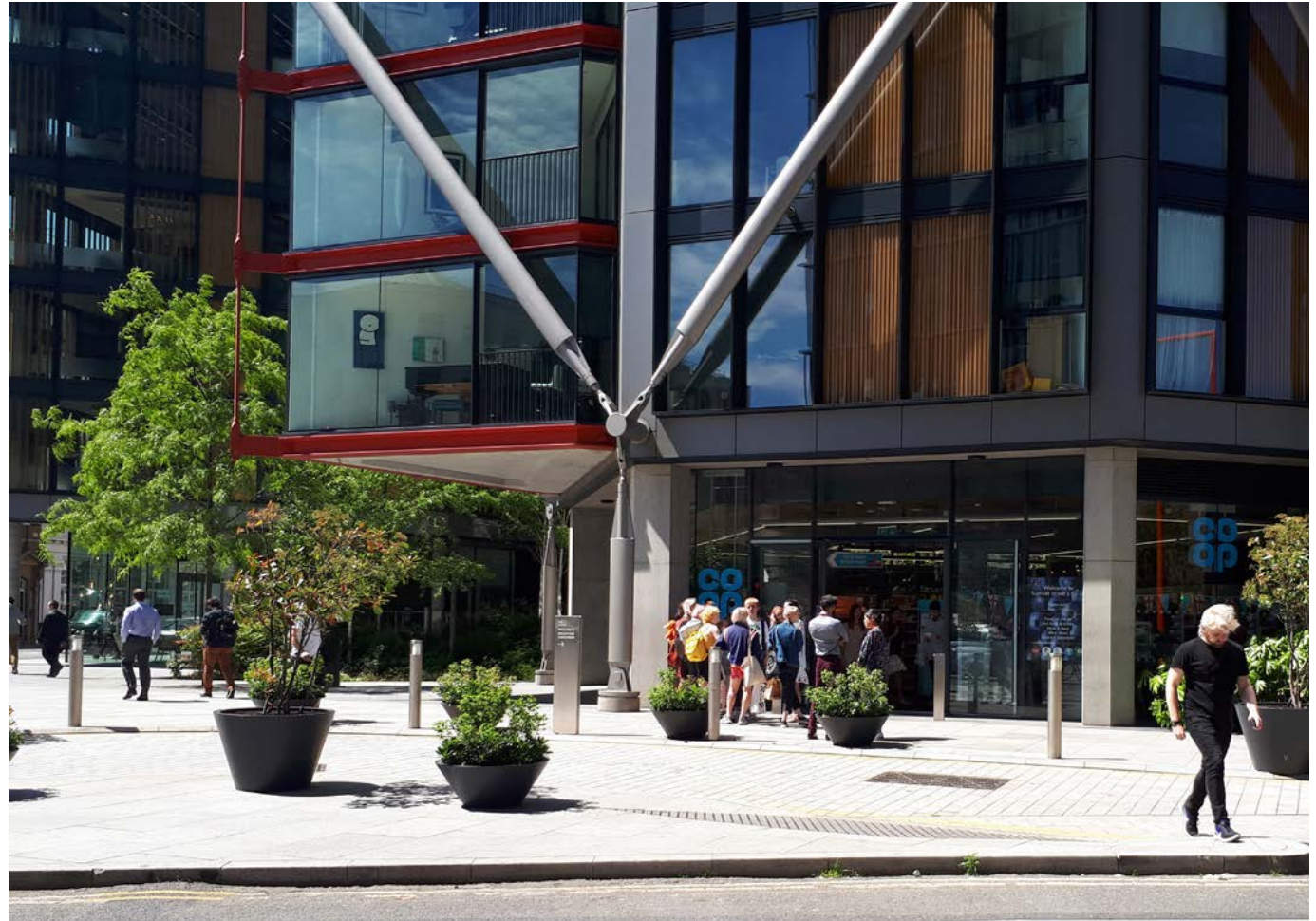
Figure 4.39: Neo Bankside, Southwark Street, London
