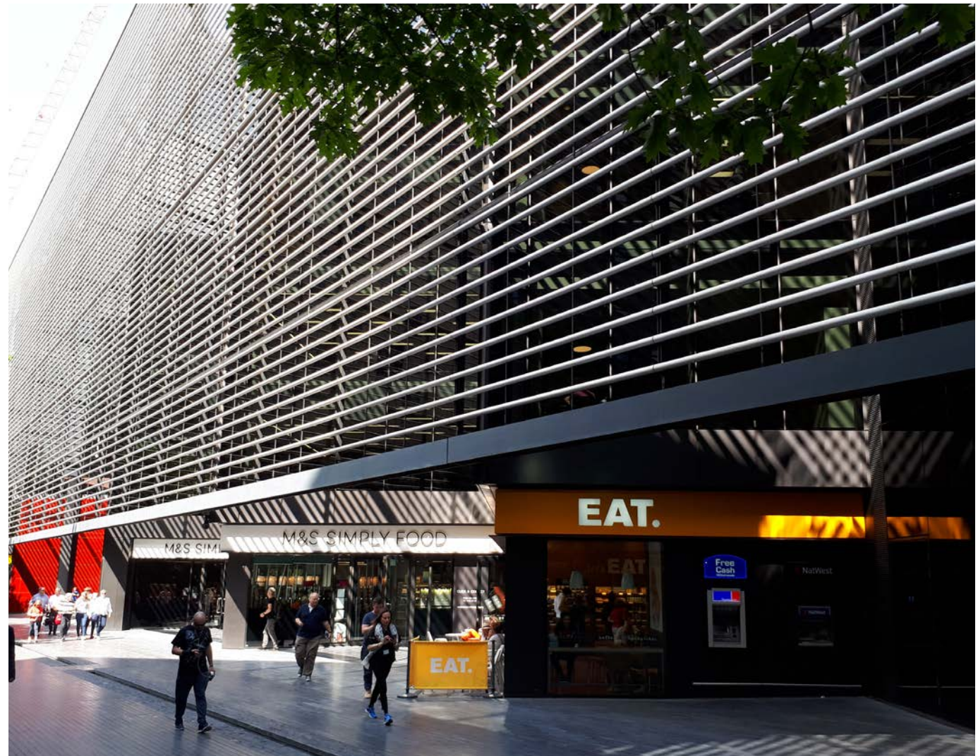
Figure 6.11: High Performance Facade, More London
