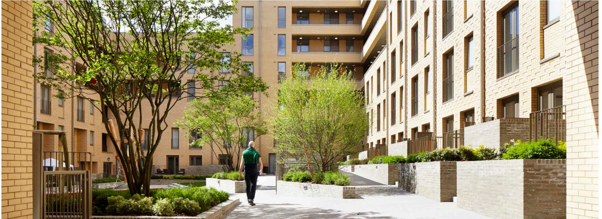
Figure 8.1: St Johns, Clapham (credit: Jack Hobhouse)
