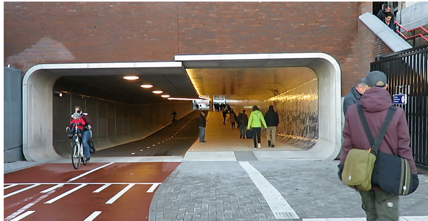
Figure 7.6: Cycle Tunnel, Amsterdam
