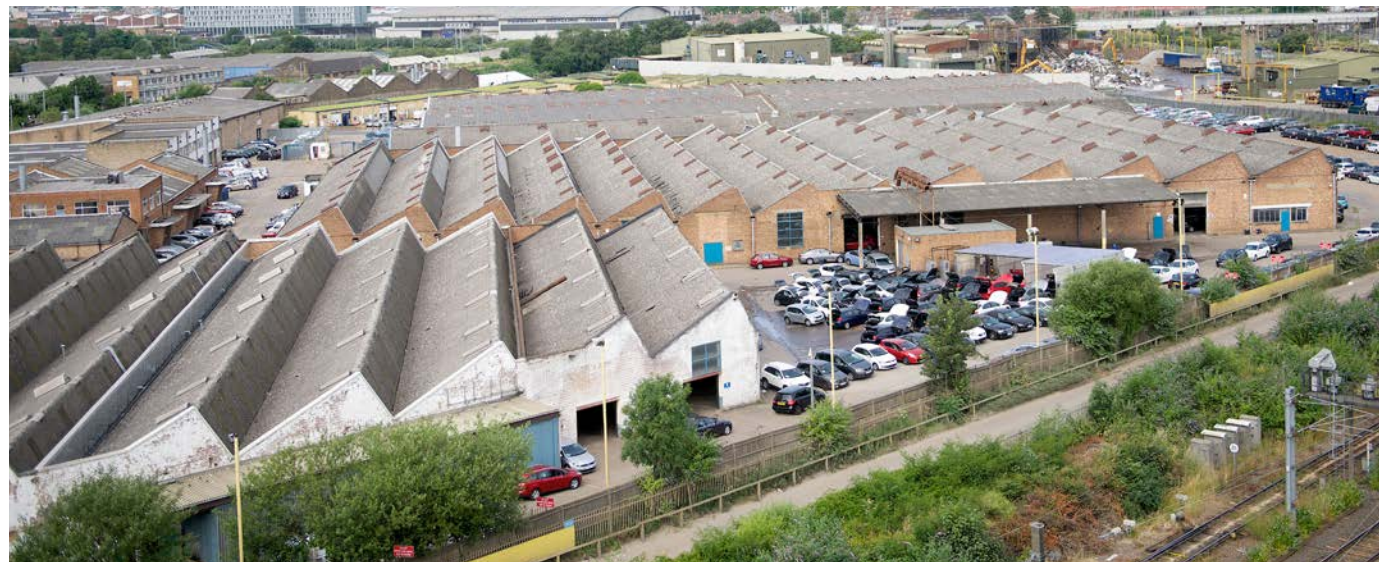
Figure 4.8: Existing industrial character of Old Oak North
