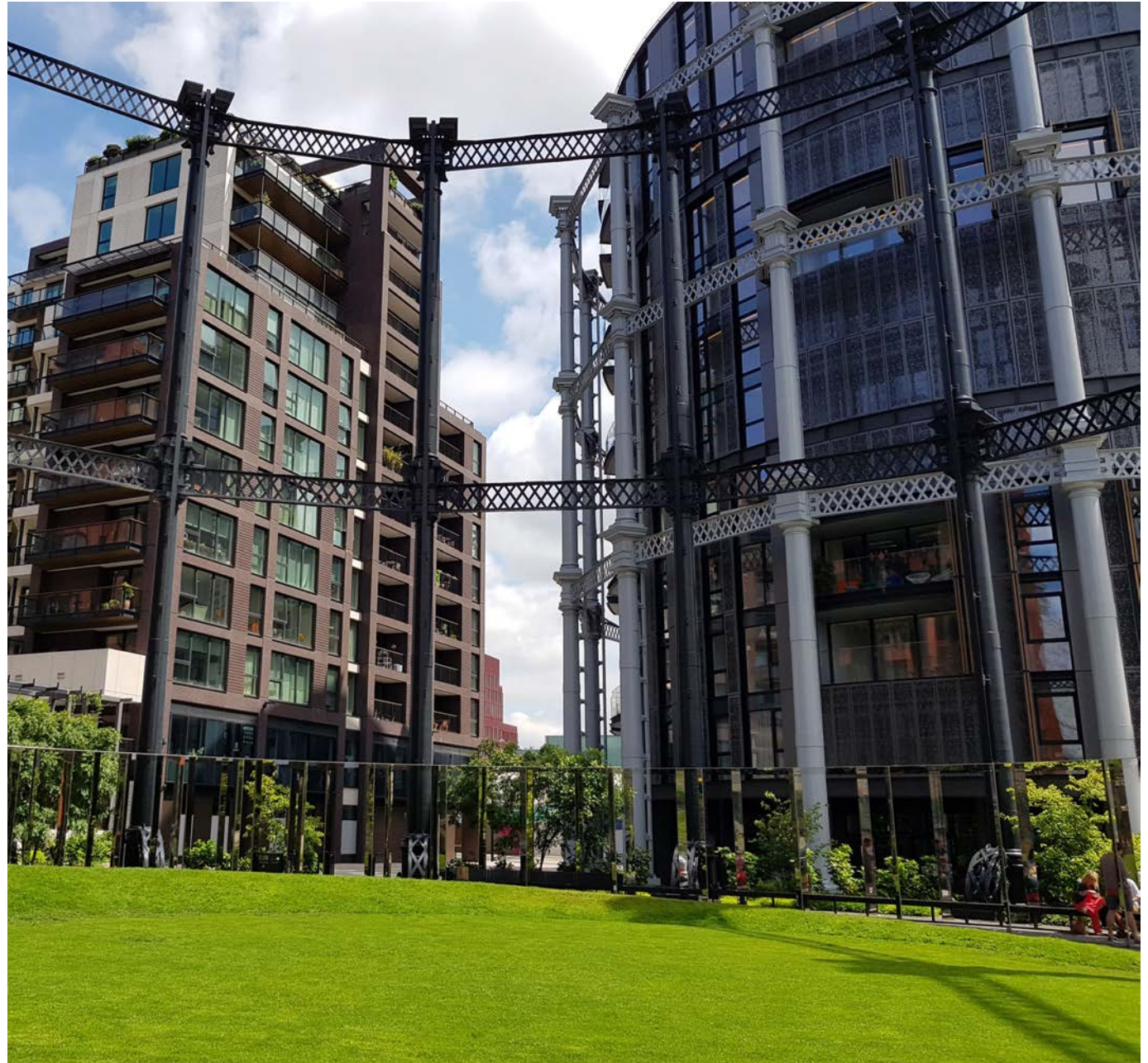
Figure 5.1: Gasholder Park, Kings Cross - precedent for delivering good growth by design and responding to local heritage
