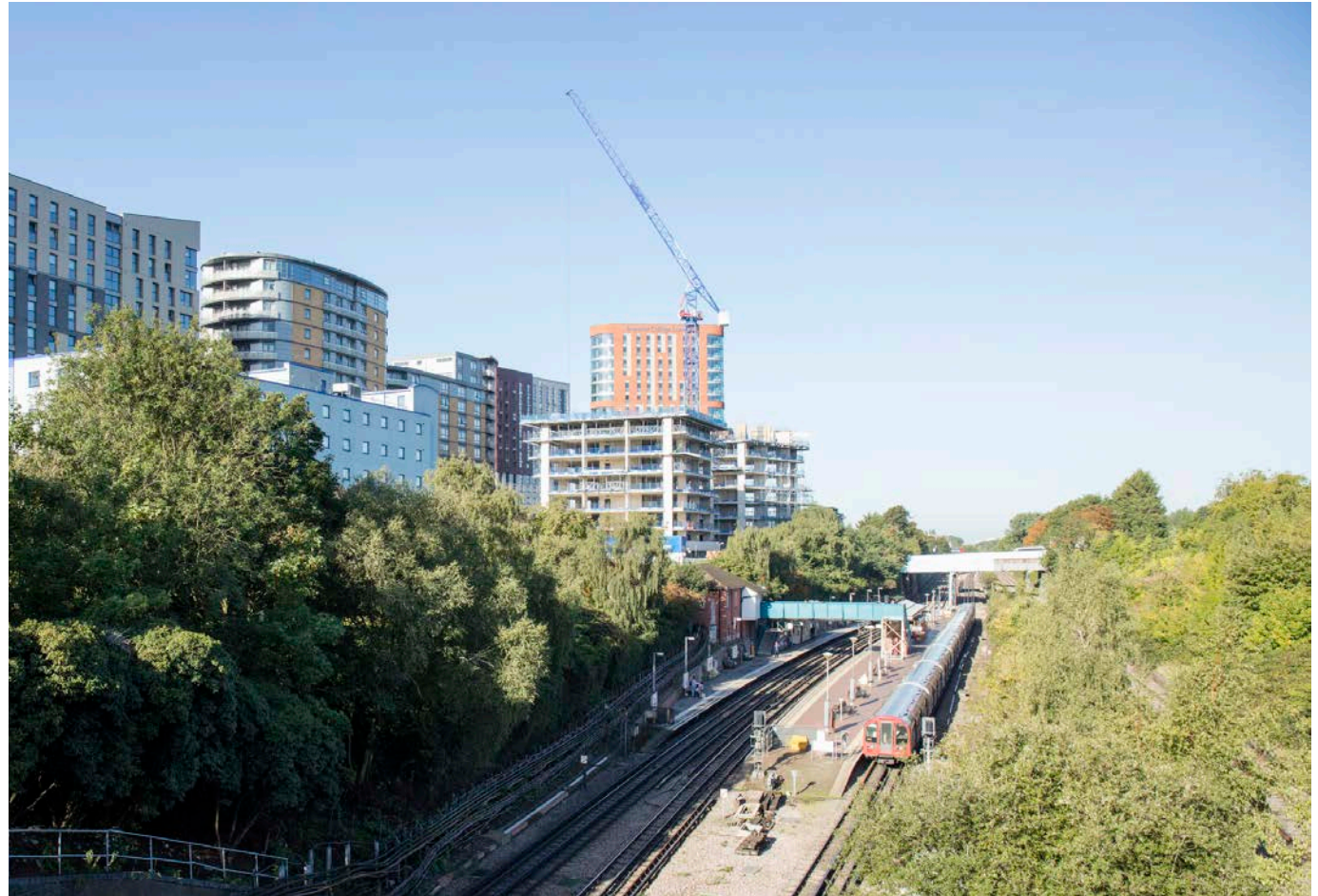
Figure 4.24: North Acton Station
