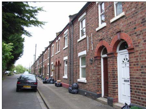
Pairs of identical houses are 'handed,' but note discord of unsuited replacement doors.
