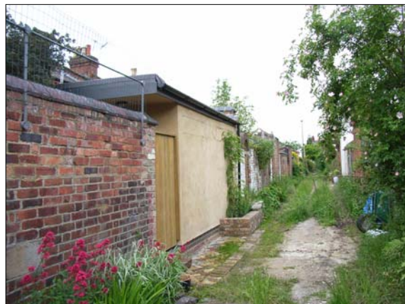
"Permitted development" such as erection of new walls and outbuildings could alter the character of back alleys unacceptably if multiplied and left uncontrolled.
