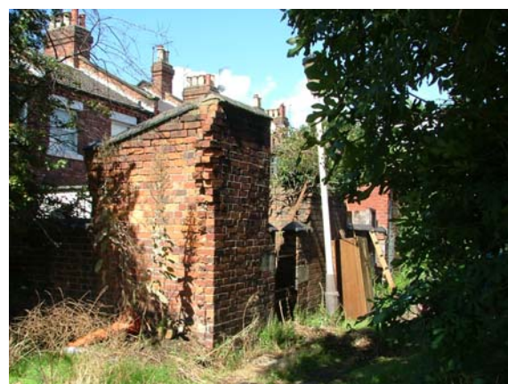
Demolition of rear boundary walls and neglect of public realm.
