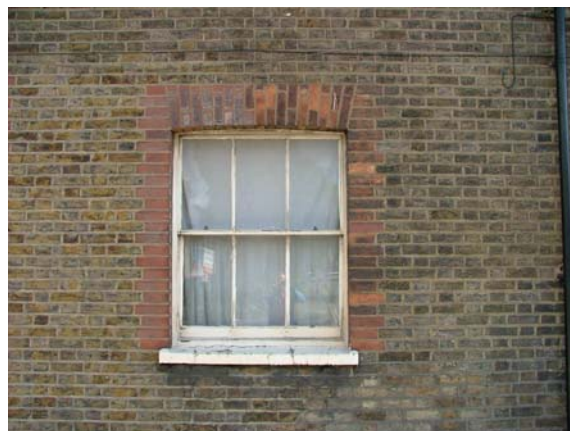
Typical brick walling, window dressing and joinery
