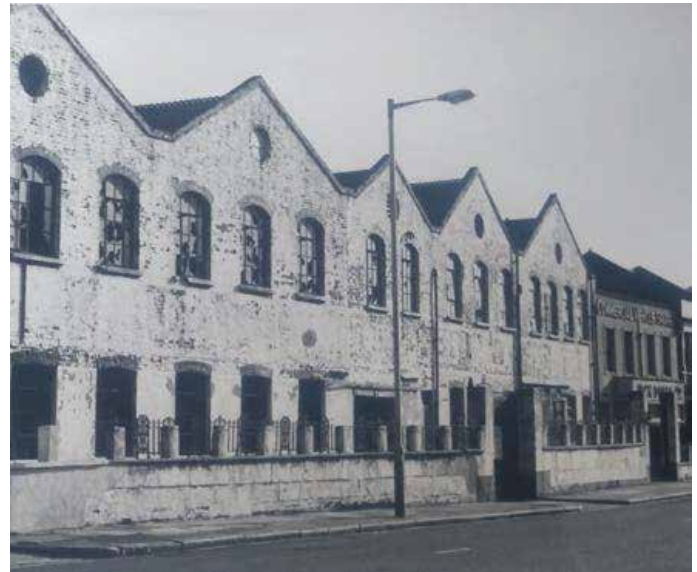
103-121 Scrubs Lane showing historic warehousing now replaced by modern equivalents
