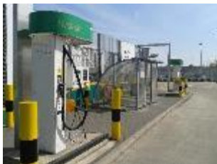
HRS at the Lea Interchange bus depot
