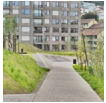
Defined edge to spray and chip surface, achieving 'clean' line to green planted edges
