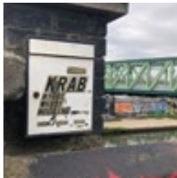
Existing post facilities at the road-level access to Mary Seacole Gardens
