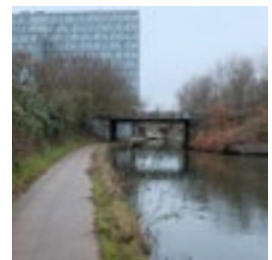
Railway bridge and immediate context evoke the canal's history
