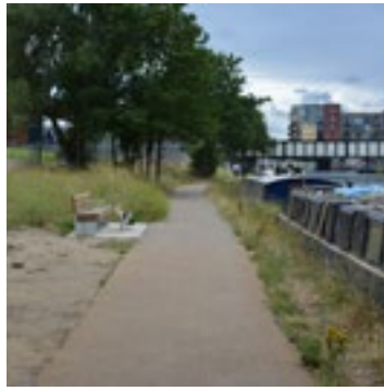
Buff spray and chip towpath with green edge and material change for bench area (Queen Elizabeth Olympic Park)
