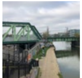
Existing bridges provide enclosure to the space and link with industrial heritage
