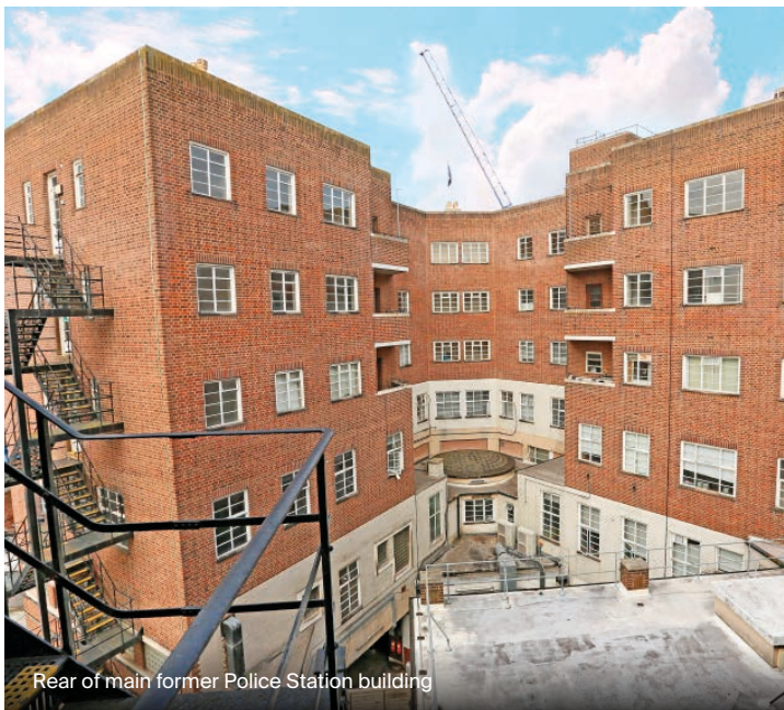
South eastern elevation of Section House building
