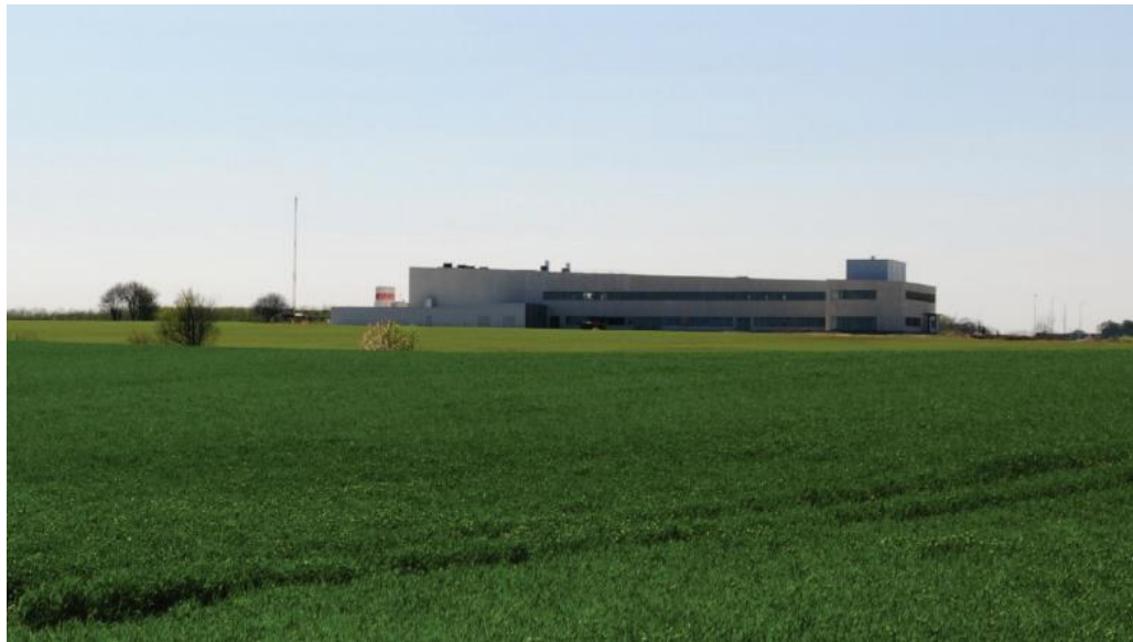
Figure 4.26 Copenhagen Clean Tech Park
