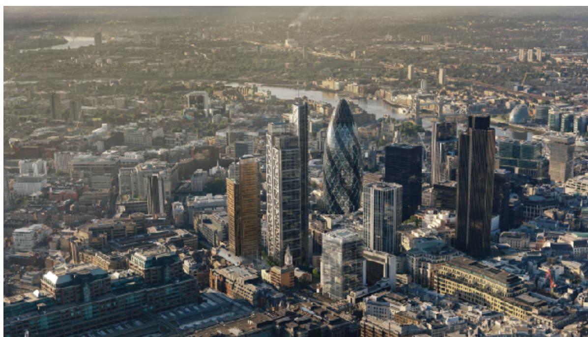
Figure 2: The proposed tower (left) looking southeast. Source: Design & Access Statement, March 2010.
