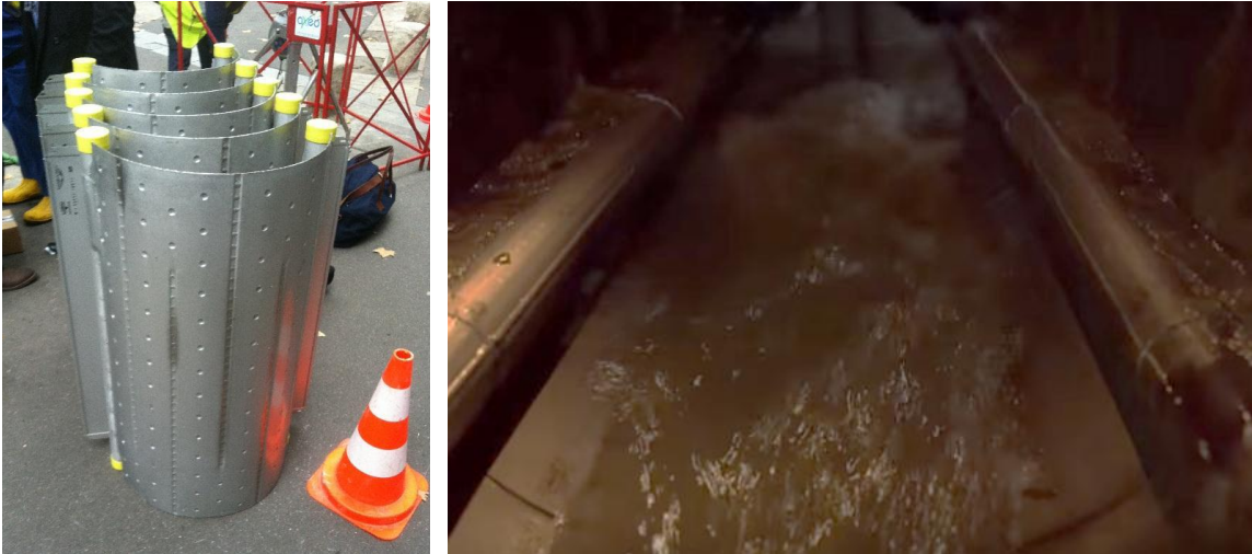
Figure A.3.5. Sewer Heat Recovery Plates Prior to Installation (left), and In Situ (right)
