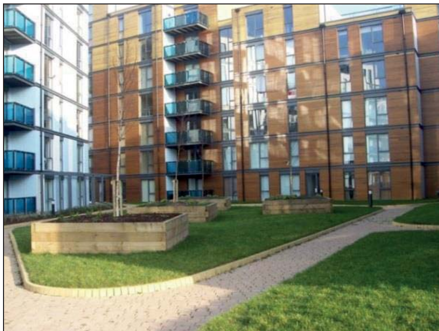
Figure 58. Permeable Paving and Landscaping over a Permavoid System on a Podium Deck
