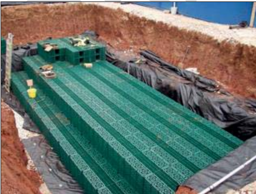
Figure 60. Underground Cellular Storage Tank
