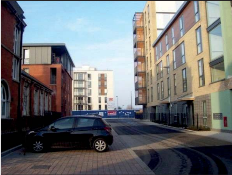
Figure 59. Permeable Paving within Car Parking Bays
