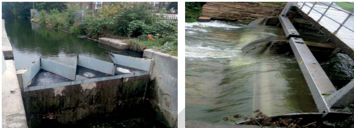
Figure 57. Crenulated and Tilting Weir Structures
