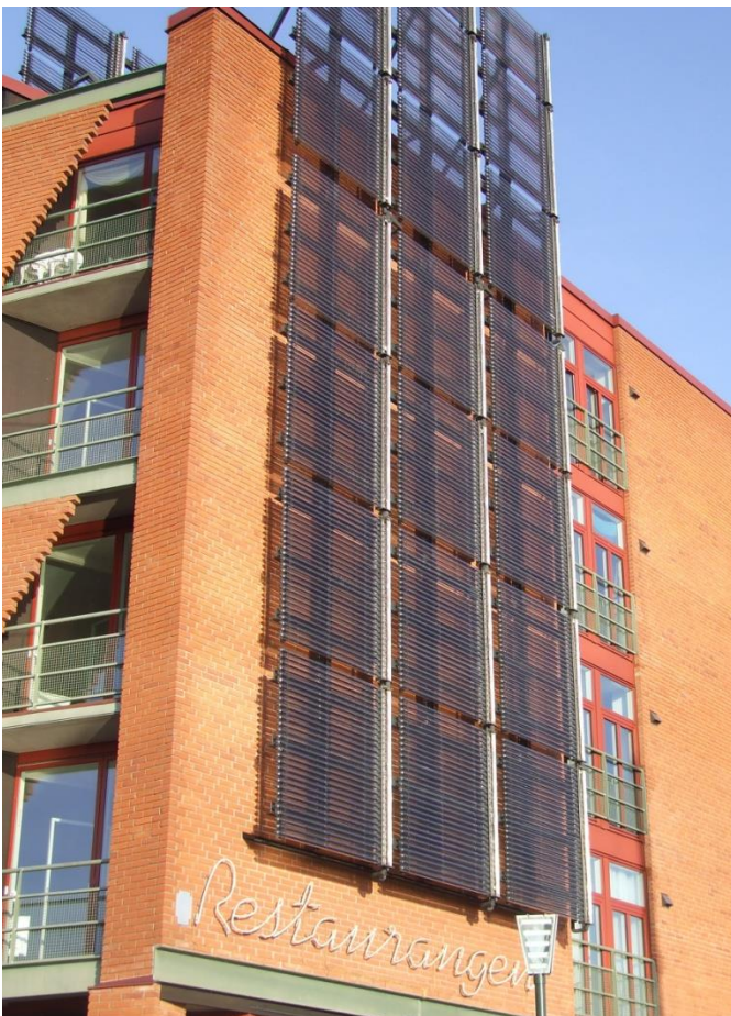
Figure A.2.3. Evacuated Tube Solar Thermal Collectors on Unshaded Façade (Western Harbour, Malmö, Sweden)
