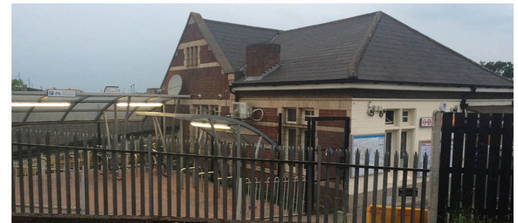
Existing Harrow Road Ticket Hall
