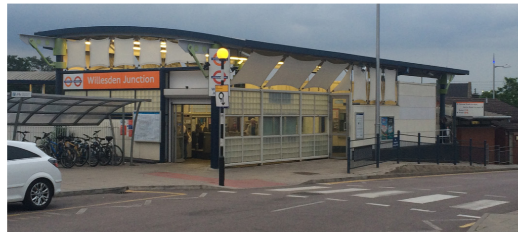
Existing Station Approach Ticket Hall
