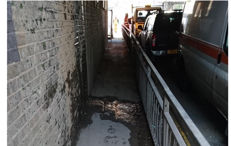
Figure 4-8: Narrow footways in railway tunnels (L17)
