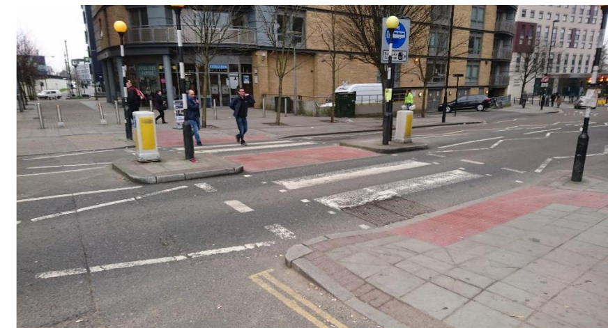
Figure 4-27: High capacity zebra crossing (C16)
