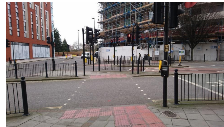
Figure 4-32: Triple staggered crossing (C18)
