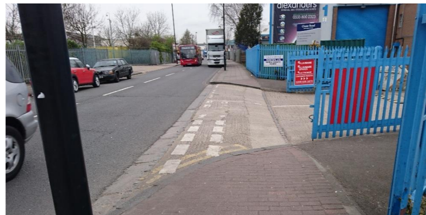
Figure 4-11: Lack of step-free access at crossovers (L20)
