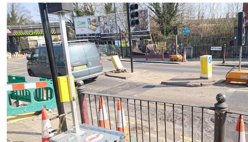
Figure 4-33: Narrow crossing at Harlesden station (C8)
