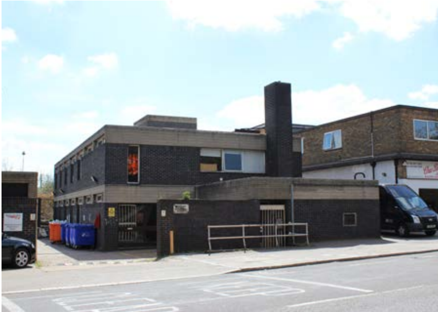
Figure 24: Willesden Junction Maintenance Depot, Old Oak Lane, a 1960s building probably designed by the British Railways Western Region Architect's Department (P6846013).
