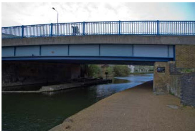
Figure 15: Ladbroke Grove Bridge, with toll gauging narrows underneath. Photograph by Andrew Lewis; reproduced from www.blog.jartweb.net by kind permission.
