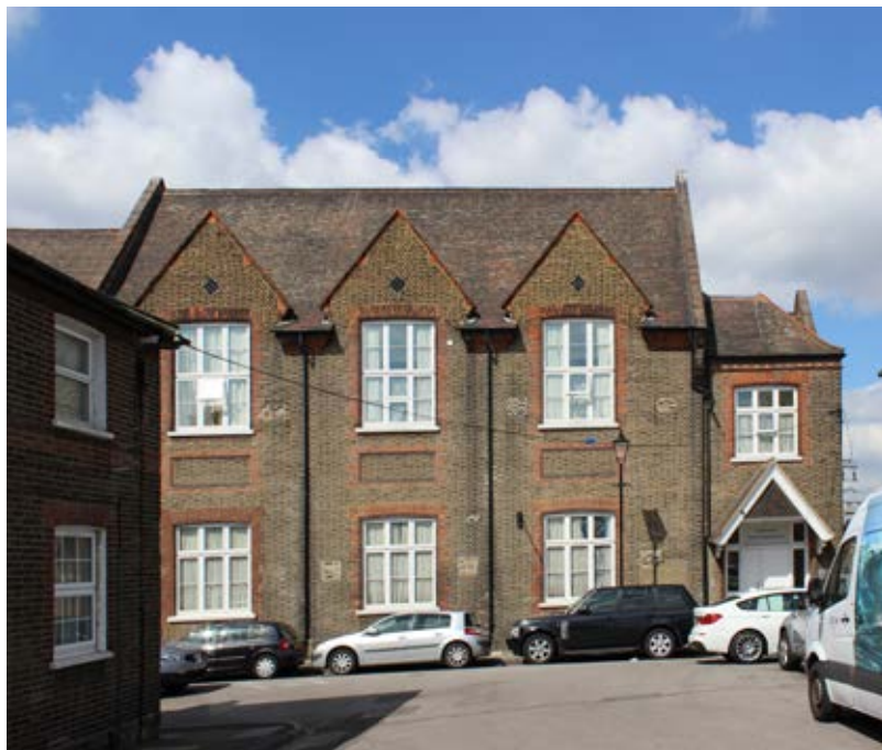
Figure 47: The former Railway Institute on Goodhall Road (P6846026).
