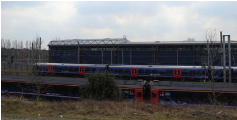
Figure 20: A view of the Eurostar maintenance shed of 1991-92 at North Pole International Depot (P6846009).
