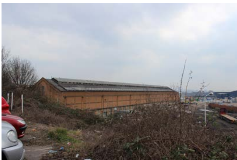
Figure 18: The carriage repair depot erected between 1936 and 1941 as part of the Great Western Railway's modernisation of the Old Oak Common Sidings (P6846008).
