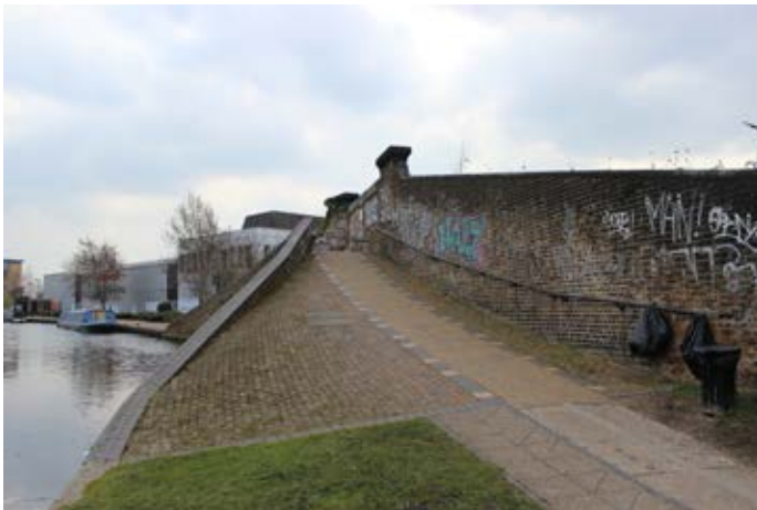
Figure 14: The humpback bridge carrying the canal towpath over the entrance to Basin No.2. Note the survival of historic surfaces and fittings (P6846006).
