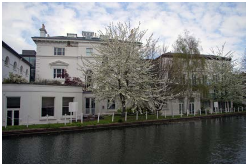
Figure 52: The stucco’d villa of c.1835, known as Kensal House, photographed from the towpath of the Grand Union Canal. Photograph by Andrew Lewis; reproduced from www.blog.jartweb.net by kind permission.
