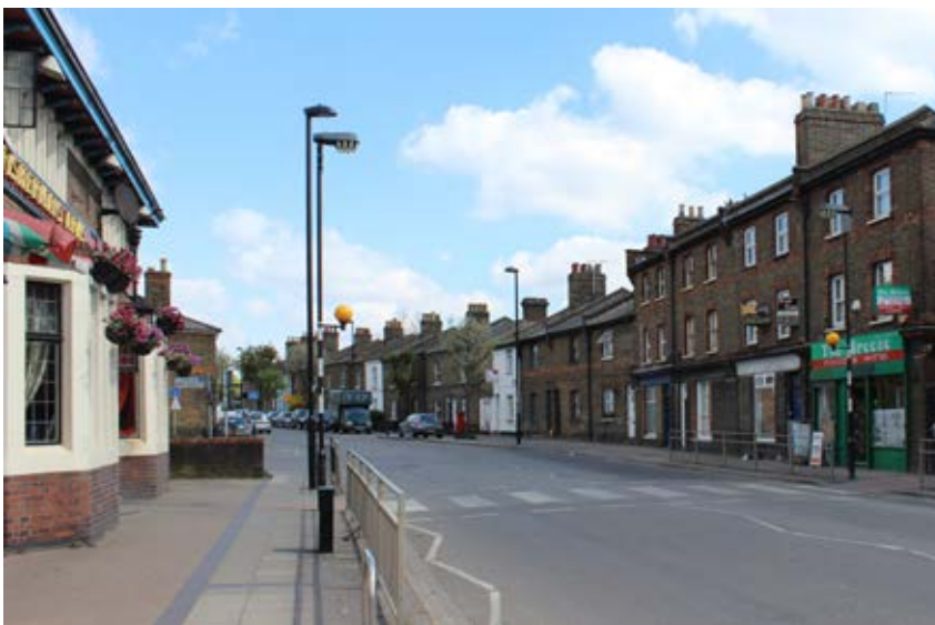
Figure 8: A view of the Old Oak Lane Conservation Area. On the left is the Fisherman's Arms, an inter-war public house (P6846004).
