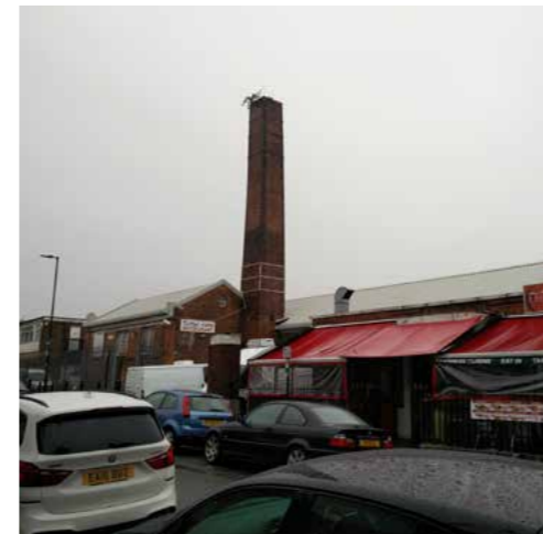
Chimney, part of the Acton Business Centre on School Road, could be incorporated into future development proposals. The building is an example of 1930s manufactory and is of local heritage interest.
