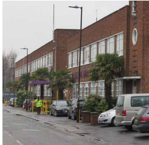
Kolak Foods Ltd. building at 308 Elveden Road, recommended for local listing
