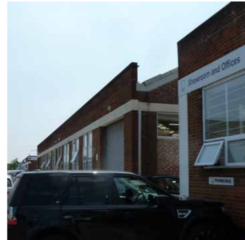
There are a number of original red-brick buildings with Flemish bond brick work, molded door casing and a brick-on-edge parapet. All the windows are replacements, and the warehouses are typical of interwar years.
