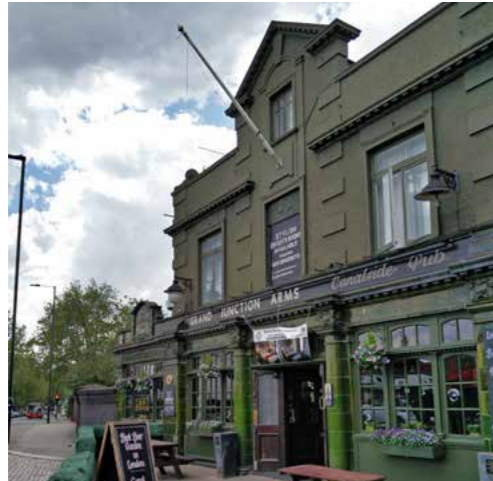
Locally listed Grand Junction Arms, elements of which date back from the original Grand Junction Railway Inn beer house of 1861
