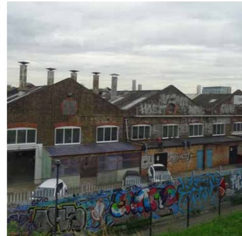
Backs of former gate and shutter works, from London Overground train
