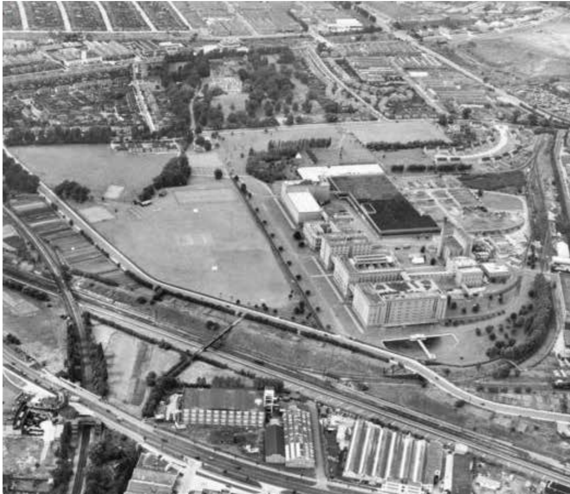
1950 aerial view west of The Guinness Brewery and environs, Park Royal. To the left is now the First Central Business Park, formerly used as a sports and recreation ground for Guinness workers. Reproduced with permission of Historic England
