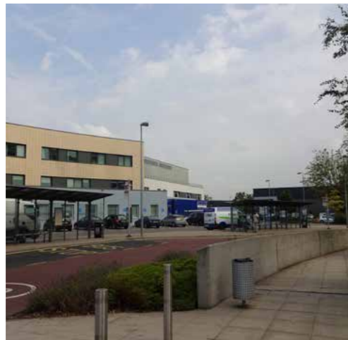
Entrance to main hospital building
