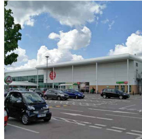
View west towards the superstore, a large free-standing rectangular building with a flat roof
