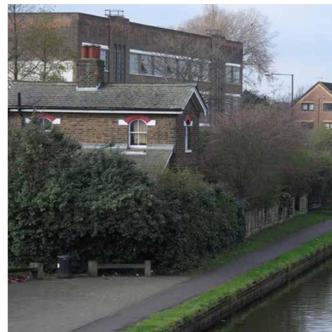
3. Willesden Junction electricity sub-station, to the east of Willesden Junction station
