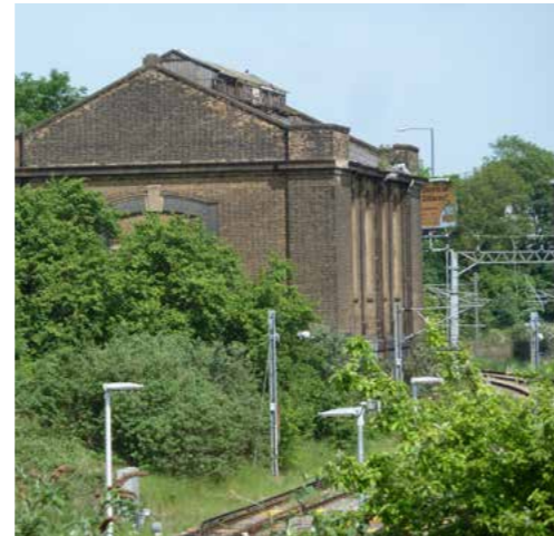
Willesden Junction electricity sub-station, built c. 1916 for the electrification of the London & North Western Railway. Large derelict brick building locally listed.
