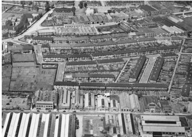
1946 aerial view north of the workers housing along Wesley Avenue, Harold Road and Newark Crescent Reproduced with permission of Historic England
