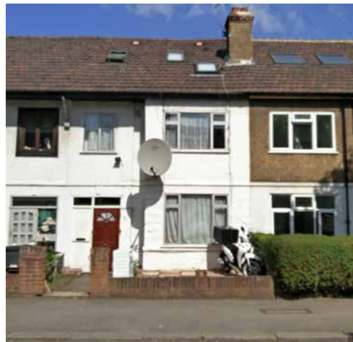
The area is characterised by blocks of terraced housing, many of which have a rough cast finish
