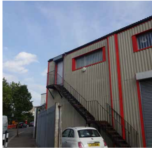
The area is characterised by warehouses with corrugated steel cladding
