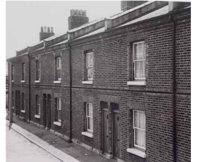
1-6 Crewe Place, Old Oak Lane, 1976 Reproduced with permission of the Hammersmith and Fulham archives
