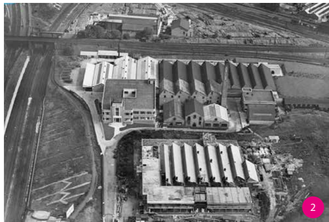
1939 Aerial image facing east showing Elizabeth Arden Factory under construction, with Monarch House and Dubilier Condenser Company behind Reproduced with permission of Historic England
