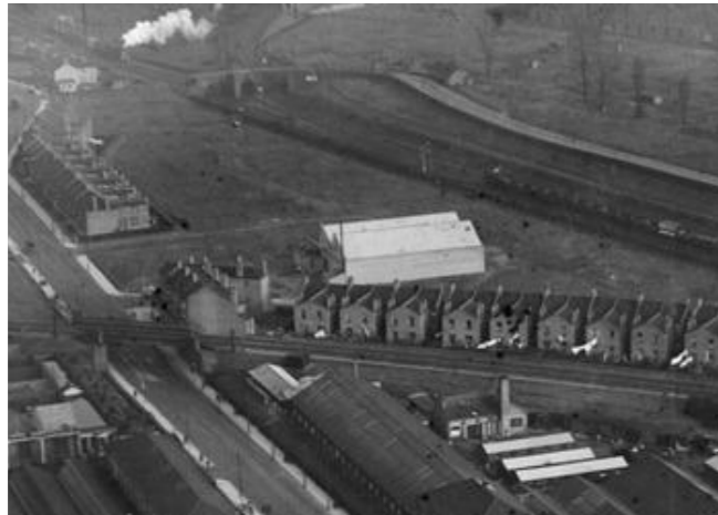
1921 view north at Midland Terrace. A row of terraces can also be seen fronting Victoria Road, demolished in 1960s. Reproduced with permission of Historic England
