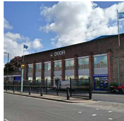
Red brick building, formerly known as 'Chase House', facade may have been retained
