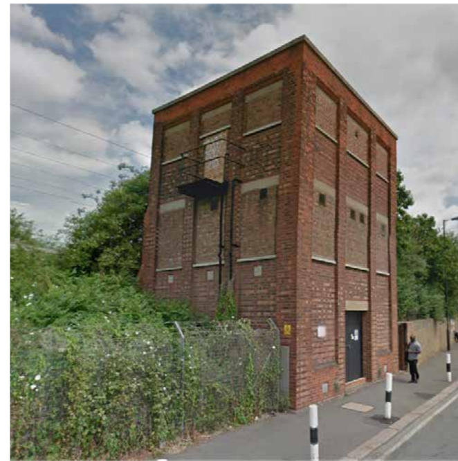
11. Electricity sub-station, Hythe Road NW10 6RT
