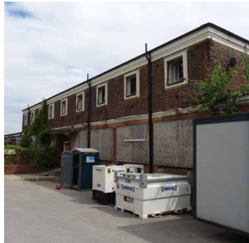
View of red brick building from Old Oak Common Lane, former British Railways Hostel
