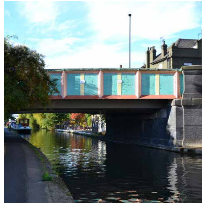
22. Acton Lane Road bridge over Grand Union Canal NW10 7NH
