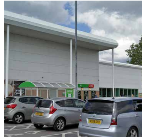
Access to the superstore favours vehicles, rather than pedestrians
