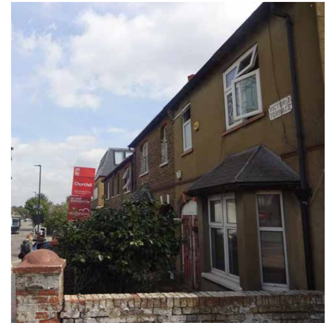
36. Victoria Terrace, 2a/b-8a/b Old Oak Lane NW10 6EG
