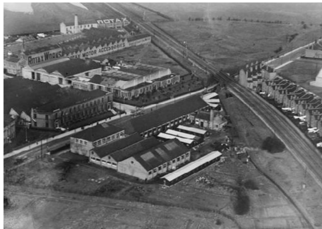
1921 aerial view of the Geographical Institute, facing north west Reproduced with permission of Historic England
