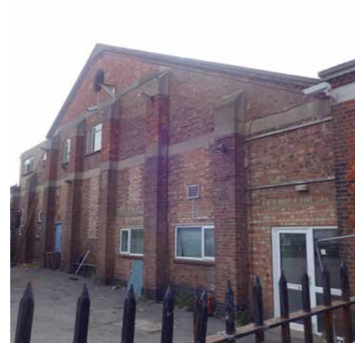
Red-brick, gable ended factory, c. 1930s
