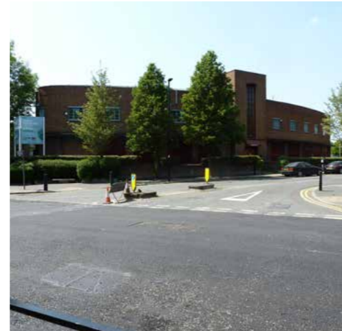
1-17 Brunel Road, a curved red brick building with art-deco influence built in the late 1920s and part of the original group of buildings that located here
