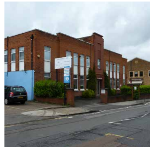
Former premises of John Compton Organ Makers, Chase Road. Rebuilt after bomb damage in the Second World War.
