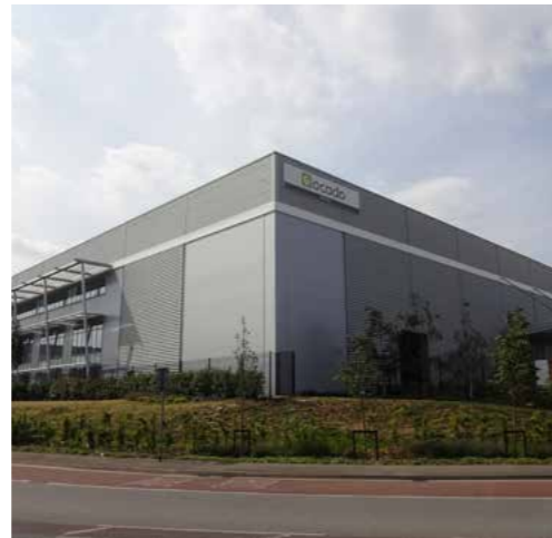
Large warehouse building to west of Rainsford Road
