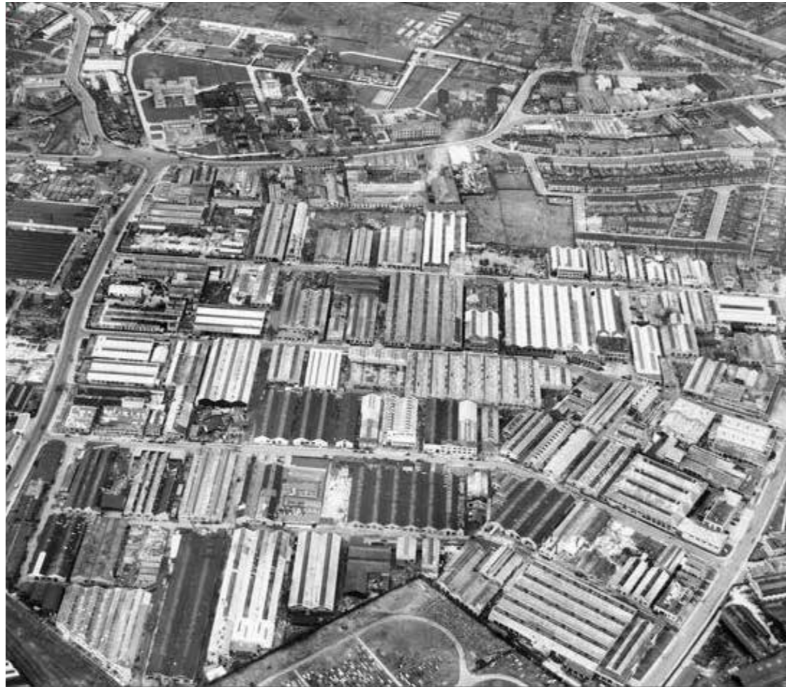
1947 aerial view looking north, showing Gorst Road and the surrounding industry in the area. Reproduced with permission of Historic England
