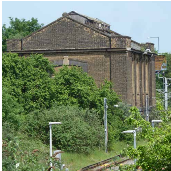
33. Willesden Junction electricity sub-station, to the east of Willesden Junction station
