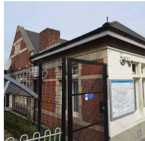
Former Willesden Junction ticket office, constructed in c.1912 and recommended for local listing
