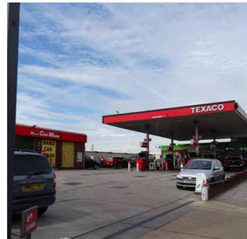
View of petrol filling station looking west along Harrow Road
