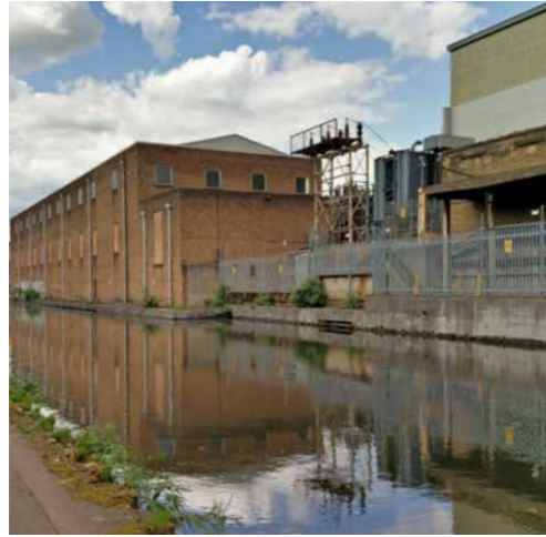
Acton Lane Power Station with dry dock
