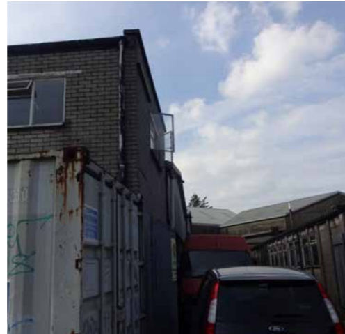
Alleyways to the back of buildings allow access for servicing
