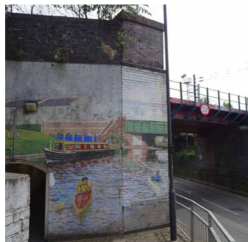
Painted murals on west wall of railway bridge crossing over Hythe Road, depicting the Grand Union Canal
