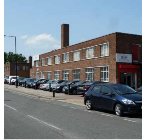
View west along Coronation Road, the brick chimney a positive feature of the streetscape
