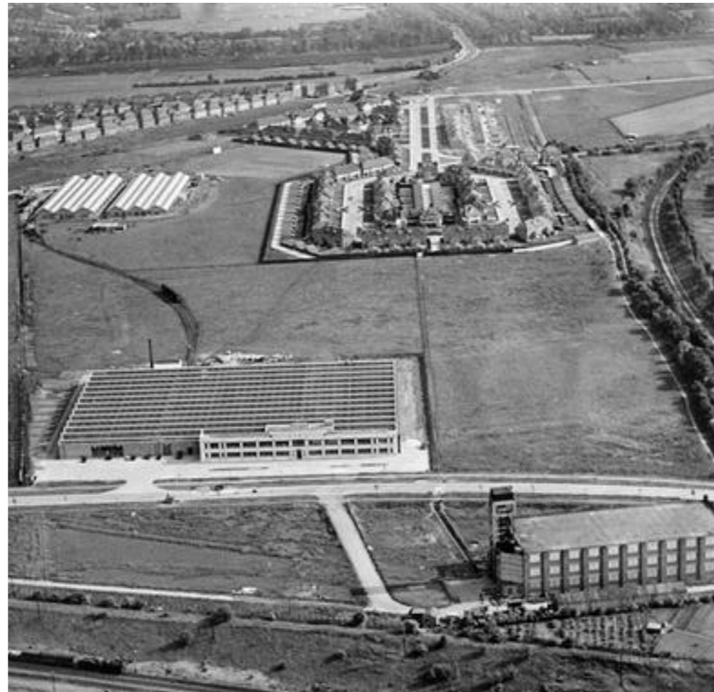
1930 aerial view of Superity House, a milk distribution factory, looking south. Primrose Gardens can be seen in the background. Reproduced with permission of Historic England
