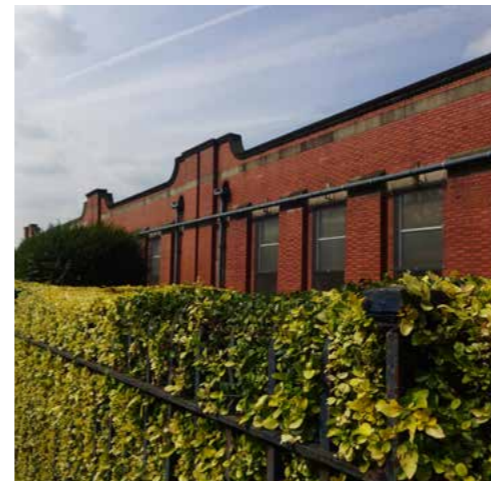
McVities building, c. 1930s, the only historic survivor from McVities biscuit works. Dates back to 1930s, should be considered for local listing
