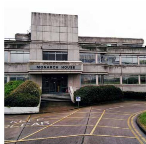
Monarch House, Victoria Road Estate, an example of c. 1970s concrete brutalist style architecture
