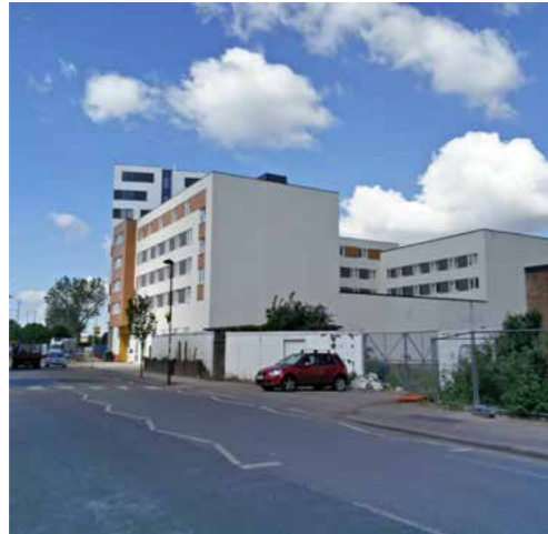
Victoria Care Centre, Acton Lane
