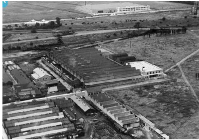
1930 aerial view south of the Mono Service Containers factory and surrounding industrial units Reproduced with permission of Historic England
