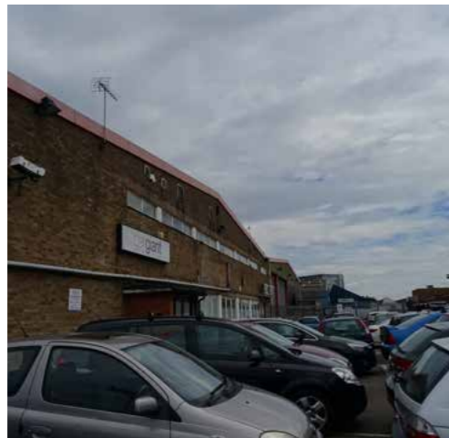
View of the Car Giant service centre on Salter Street, tarmac and concrete surfaces dominate the area
