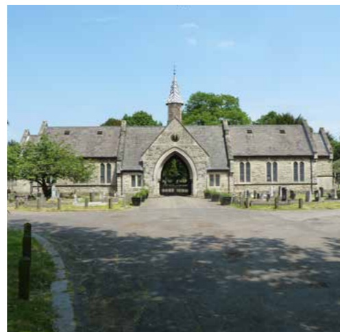
The two chapels at the southern entrance to the cemetery were constructed at the same time as the cemetery was laid out in 1895 and are recommended for local listing
