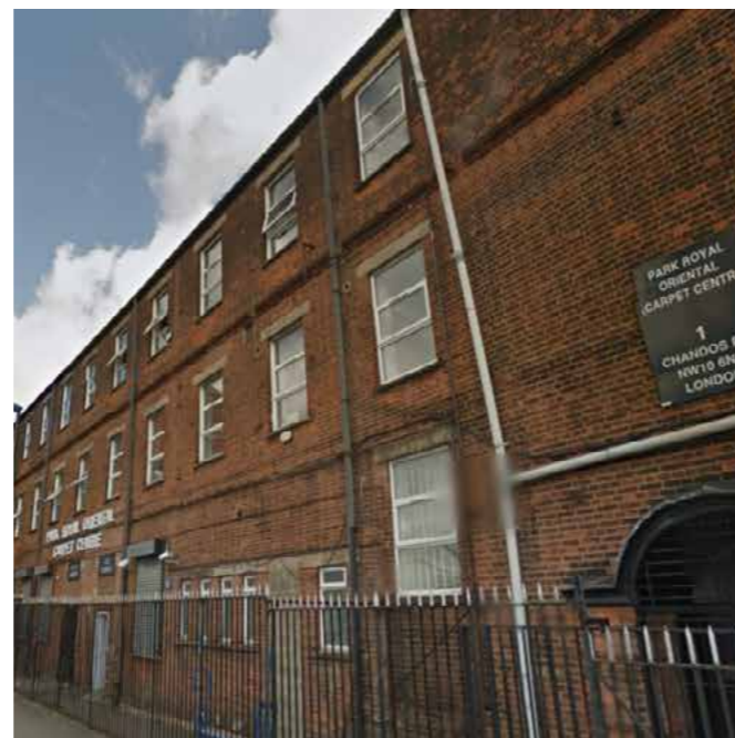
6. Former Rotax Works, 1 Chandos Road NW10 6NF
