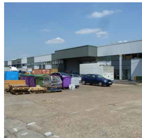
View of large warehouse buildings with corrugated steel cladding to the east of Dukes Road
