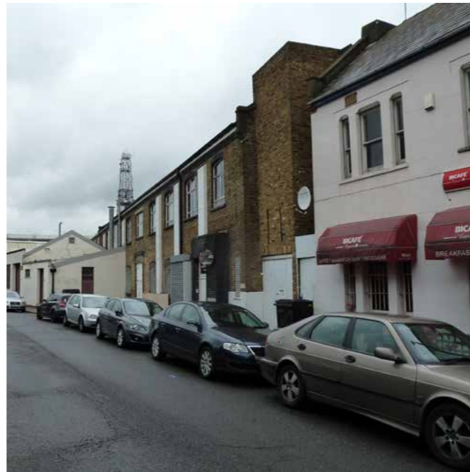
10. Former Engineering Works, 18-19 Hythe Road, NW10 6RT
