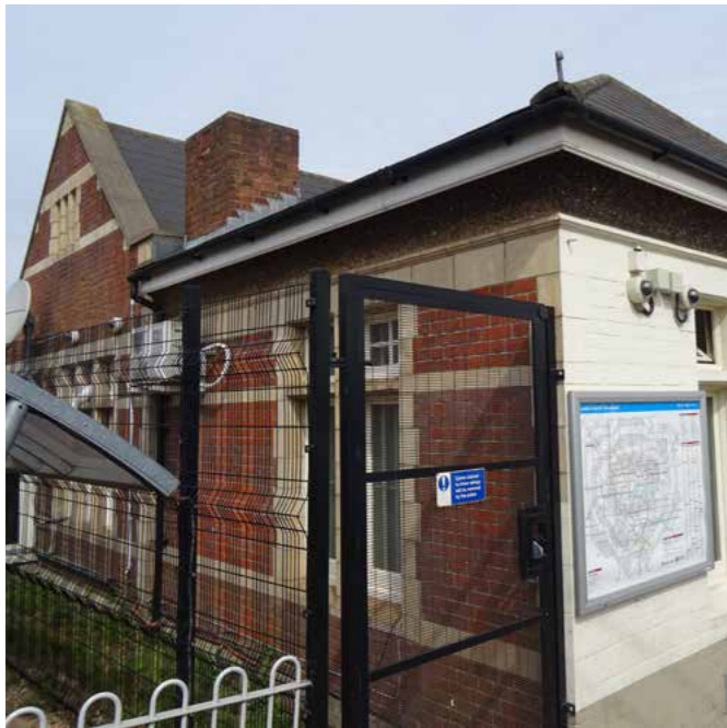
17. Willesden Junction former ticket office (Harrow Road entrance), NW10 4UY
