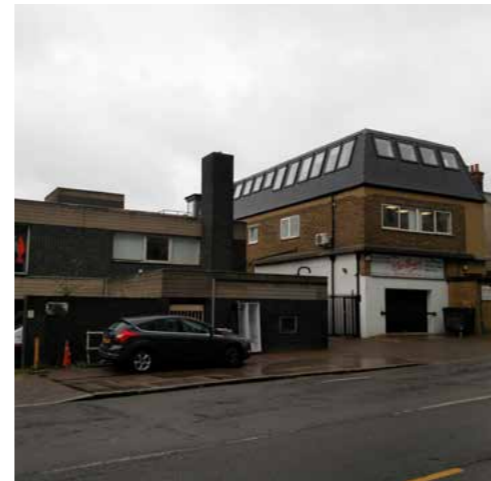
A small number of single free-standing buildings were constructed in a piecemeal fashion in the mid 1900s to the south of Old Oak Lane adjacent to Victoria Terrace
