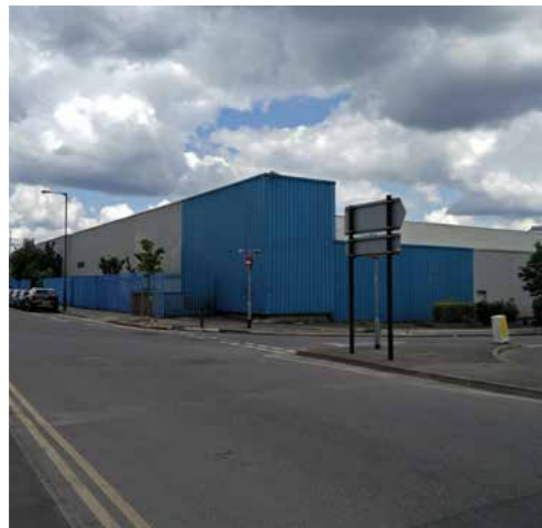
Large warehouse on corner on Rainsford Road and Whitby Avenue
