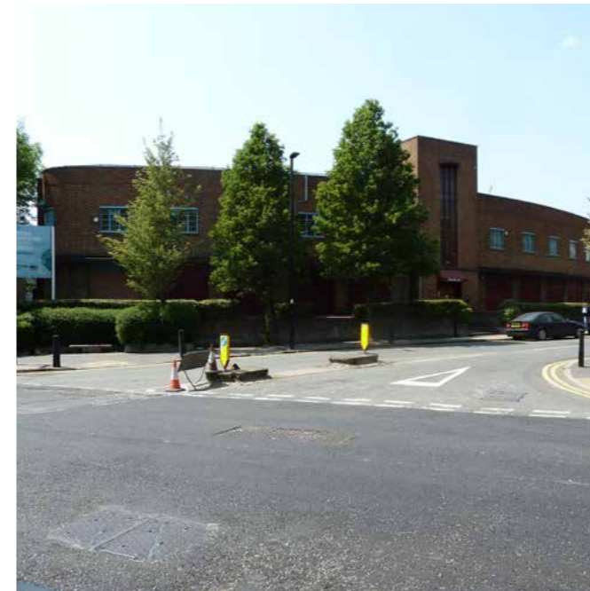
15. 1-17 Farley building, Brunel Road W3 7XR
