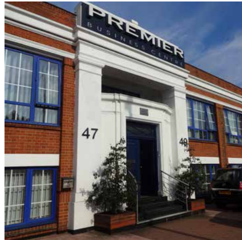
47-49 Park Royal Road, building of significant heritage interest
