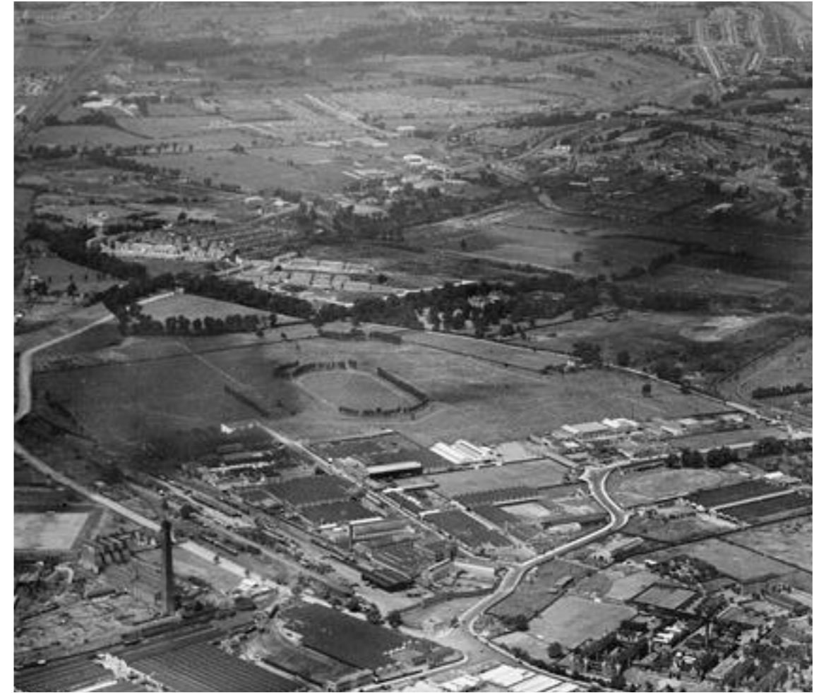
1933 aerial view of the Horse Ring and various factories from the south-east. Abbey Road is the curving road to the bottom right and Cumberland Avenue is the road in the centre of the image. Coronation Road is to the bottom left Reproduced with permission of Historic England
