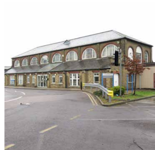
The Old Refectory on Central Way, two storeys with stock brick and red brick dressings with a hipped slate roof
