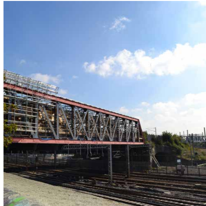
30. West London line overbridge NW10 6QE
