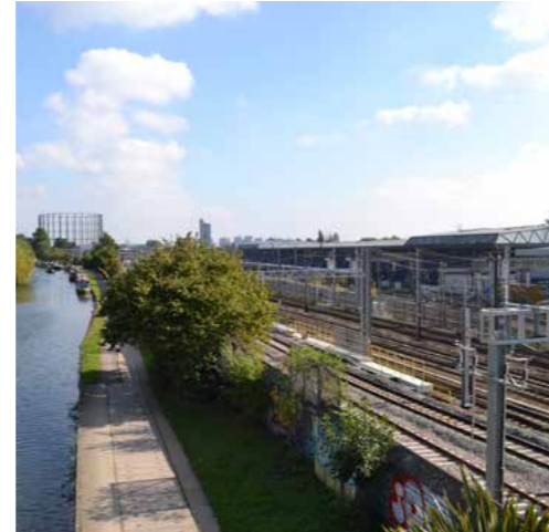
View looking east from Mitre Bridge, the Great Western Railway lines run adjacent to the canal
