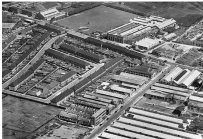
1946 aerial view looking east, showing housing laid out for Harold Wesley employees Reproduced with permission of Historic England
