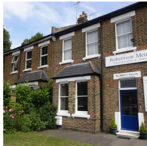
Brett's Villas, a late Victorian symmetrical pair of villas in stock brick with original sash windows and a hipped slate roof
