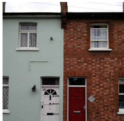
Many of the houses have been altered and differ greatly from their original appearance
