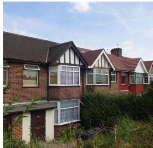
Housing along the north-side of Western Avenue, constructed c. 1930s
