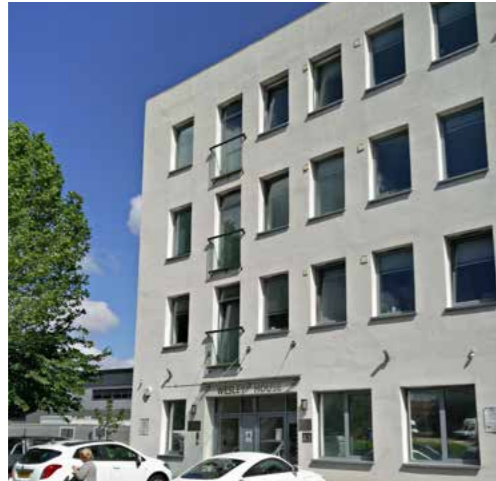
Four storey building on the corner of Wesley Avenue and Acton Lane, built post 1950s
