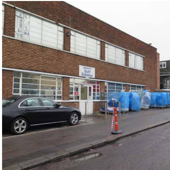
21. 304-306 Elveden Road NW10 7SY
