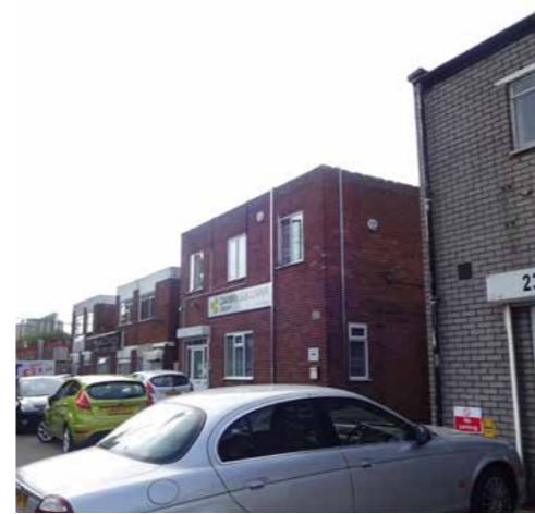
View west down Barretts Green Road showing free-standing red-brick structures
