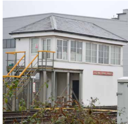
Locally listed Acton Canal Wharf signal box, built c.1895
