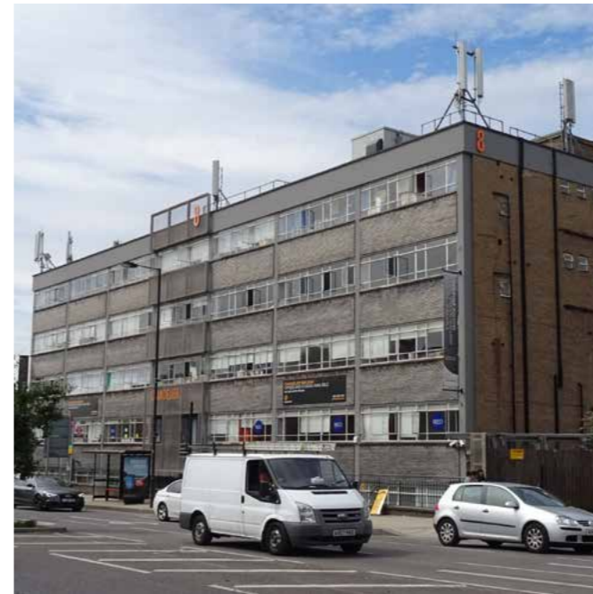
19. Chandelier building, Scrubs Lane NW10 6RB
