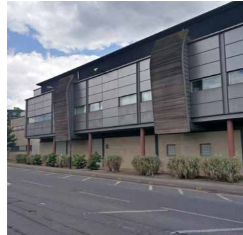
Ambulatory Care and Diagnostic Centre, Acton Lane
