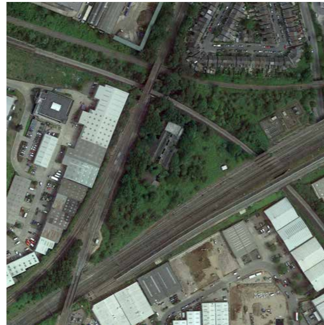
34. Electricity sub-station, south east of Wells House Road
