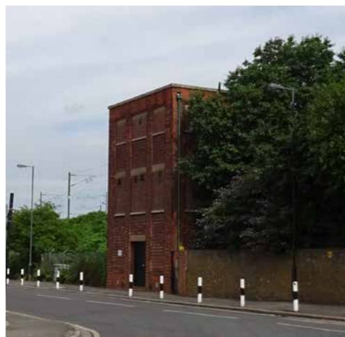
View of electricity Sub-station, Hythe Road, proposed locally listed
