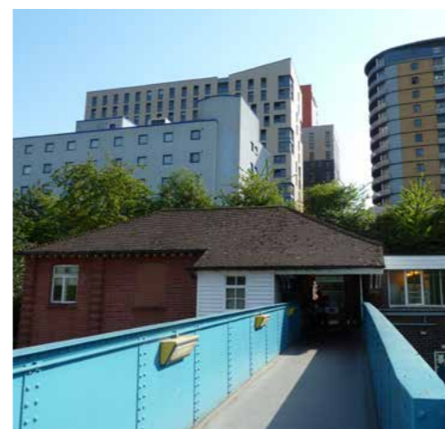
View looking south at back of North Acton Station with new developments in the background
