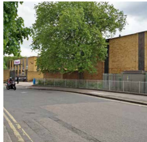
Large yellow-brick buildings along Cumberland Avenue with blank facades
