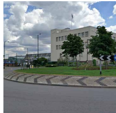
View of HMR on corner of west side of Cumberland Avenue and Rainsford Road
