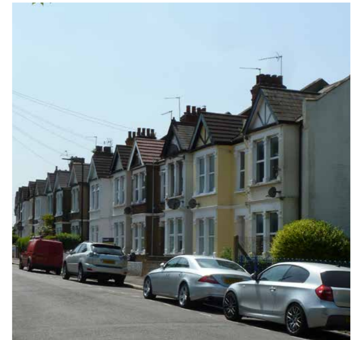
4. 4-46 (even) Midland Terrace, Victoria Road NW10 6LB
