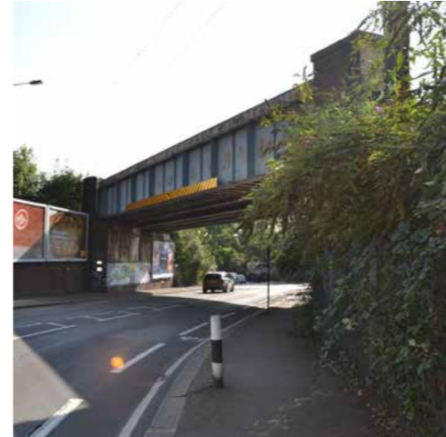
Scrubs Lane underbridge
