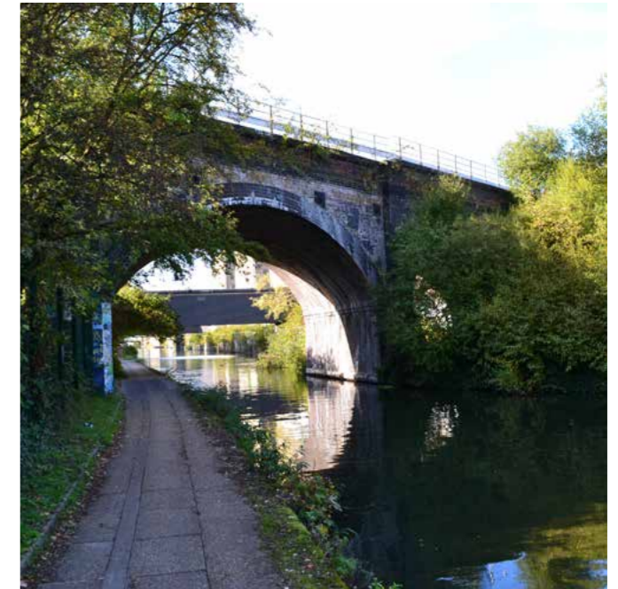
32. Railway Bridge No 8B Near Channel Gate Road
