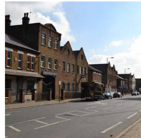
East side of Scrubs Lane, former Cumberland Park Factory, recommended for designation as a Conservation Area
