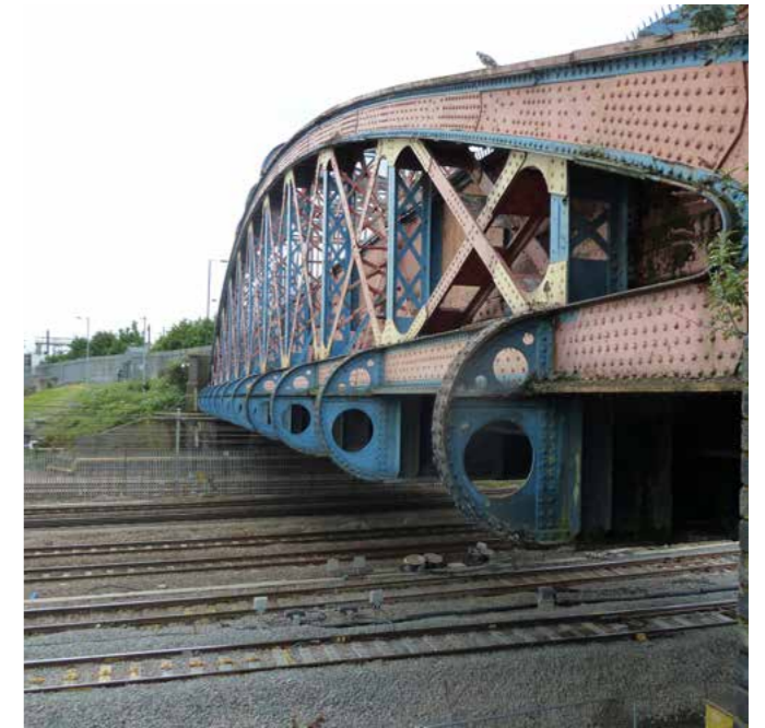
28. Scrubs Lane over bridge NW10 6QE
