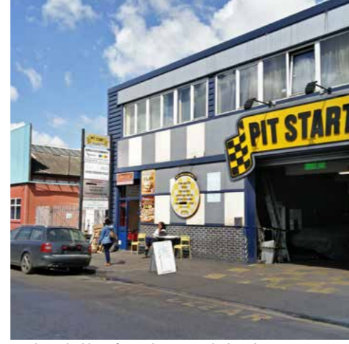
Warehouse building of neutral merit, Standard Road
