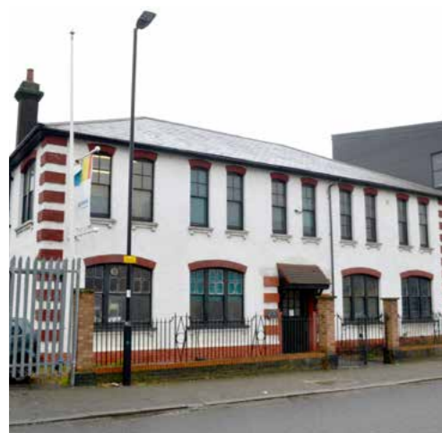
Early 20th century commercial building on St. Leonard's Road should be considered for local listing
