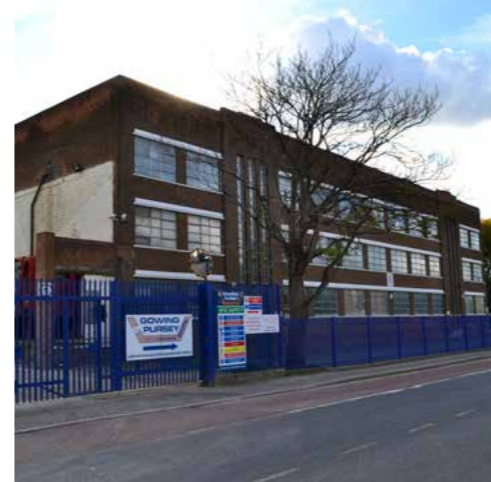
Former printworks, on the corner of Twyford Abbey Road and Rainsford Road, recommended for local listing
