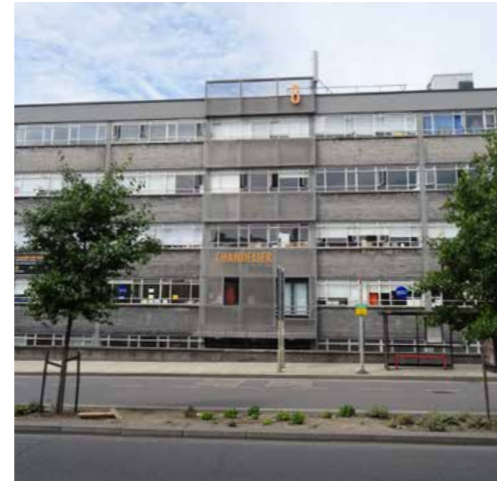
View of Chandelier building, five-storey 1960s building, of positive importance to townscape and suitable for re-use
