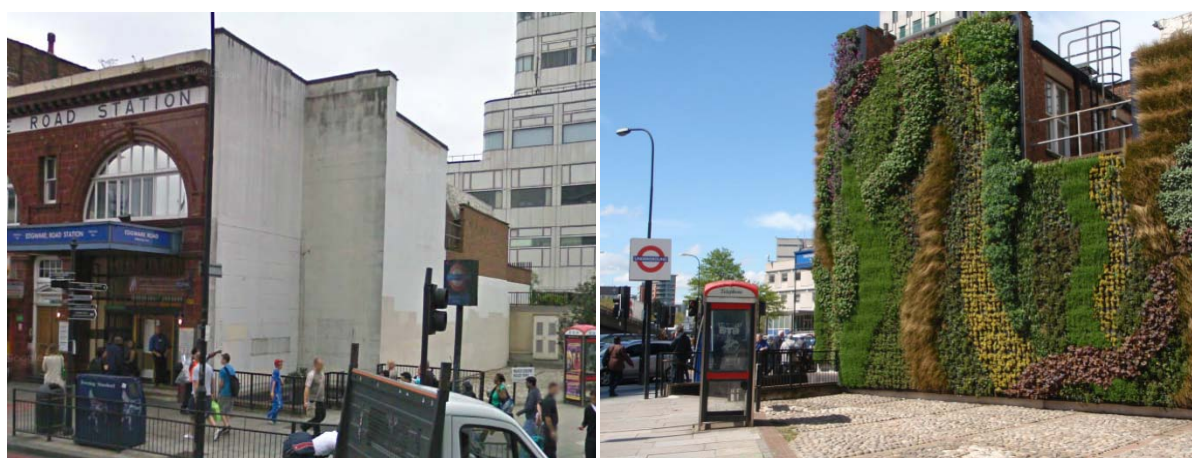
Figure 1: Edgware Road LU station before and after construction
