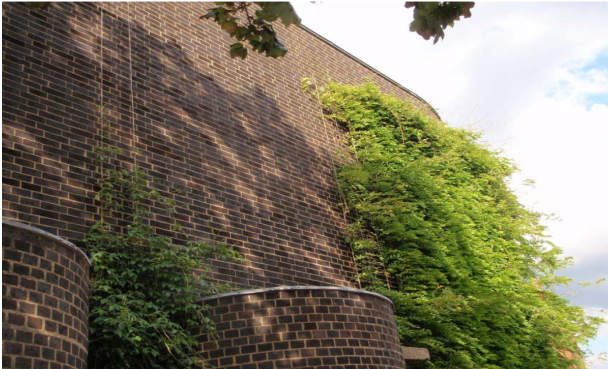
Figure 6: Green wall with self-supporting climbing plants
