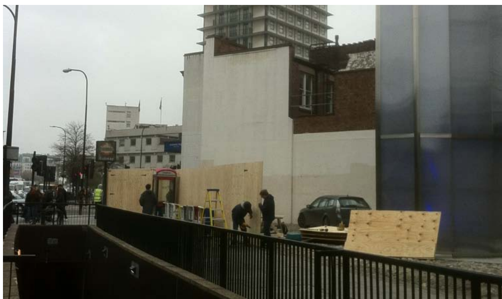
Figure 13: Showing the construction of the site compound.
