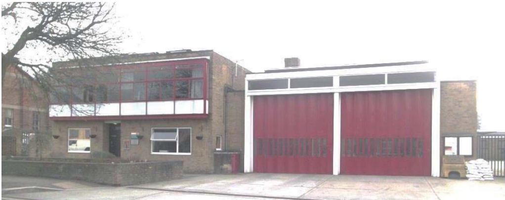
Figure 10.1 Existing Park Royal Fire Station
