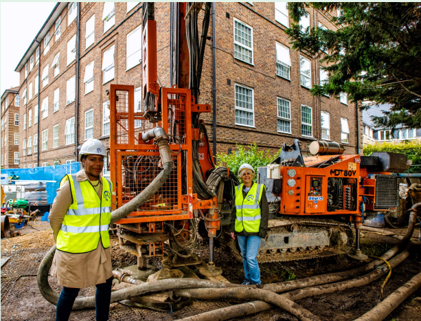
Drilling of the borehole which provides water for the heat pump
