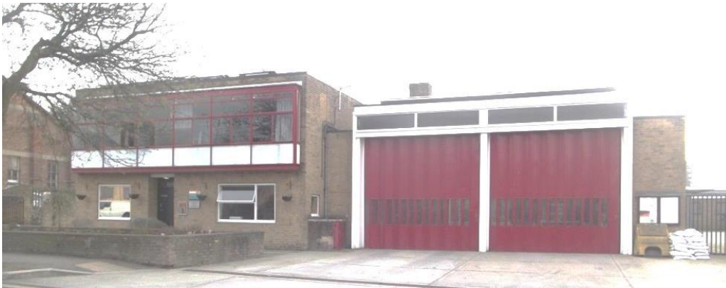
Figure 10.1 Existing Park Royal Fire Station
