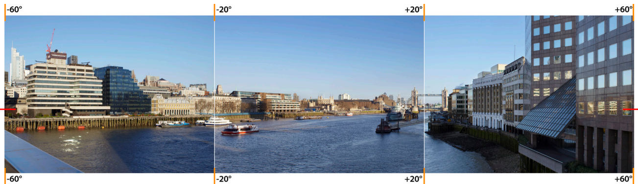
Panorama from Assessment Point 11B.2 London Bridge: downstream – close to the Southwark bank
