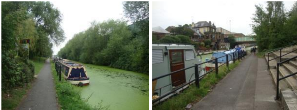
On-site evidence of low utilisation of the canal.
