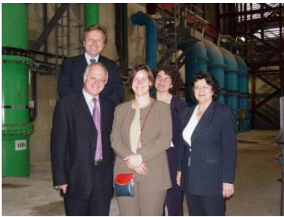
Members of the Committee at Thames Water’s Abbey Mills Pumping Station
