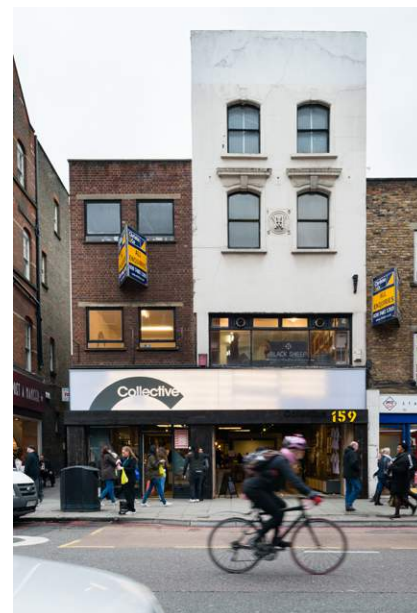
Above: Entrance to Camden Collective C/159, Camden High Street
