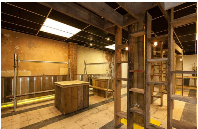
Above: C/159 pop-up retail space under construction
