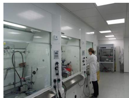
Top: Shared waste sterilisation equipment Above: Fume hood extraction facilities
