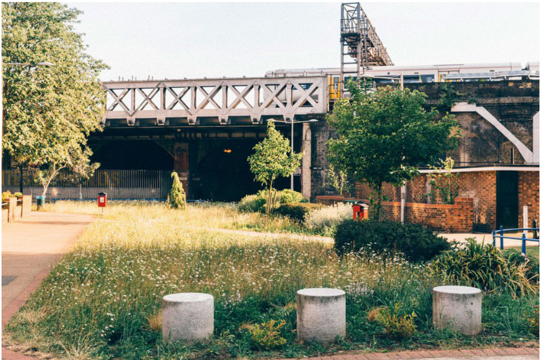
Photos of proposed arch reuse and existing green spaces, see project website
