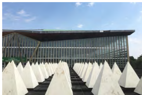
Top East elevation of the 25m pool building
