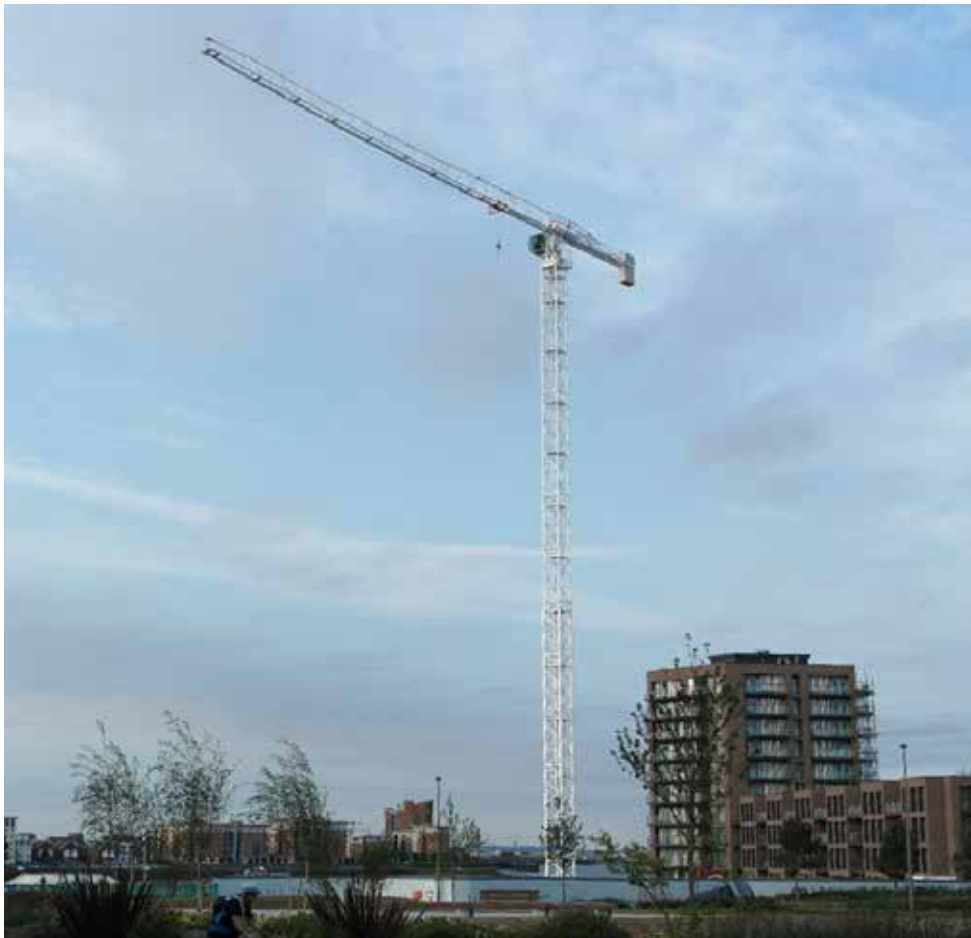
CRANE WORKING ON A THAMES DEVELOPMENT SITE, WOOLWICH
