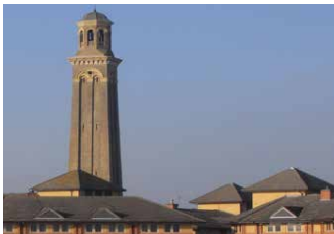
STANDPIPE TOWER AT LONDON MUSEUM OF WATER & STEAM
