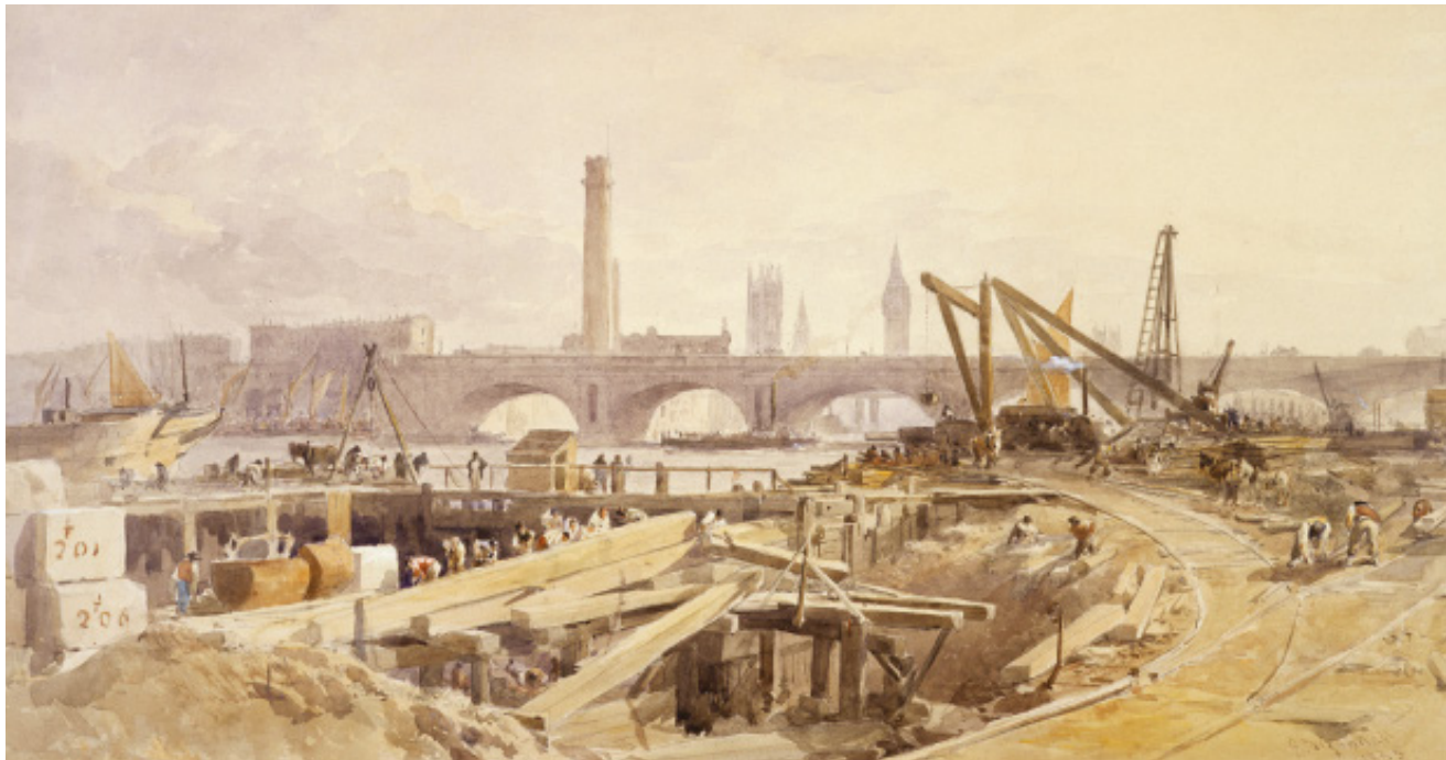
THE CONSTRUCTION OF THE VICTORIA EMBANKMENT, 1865
