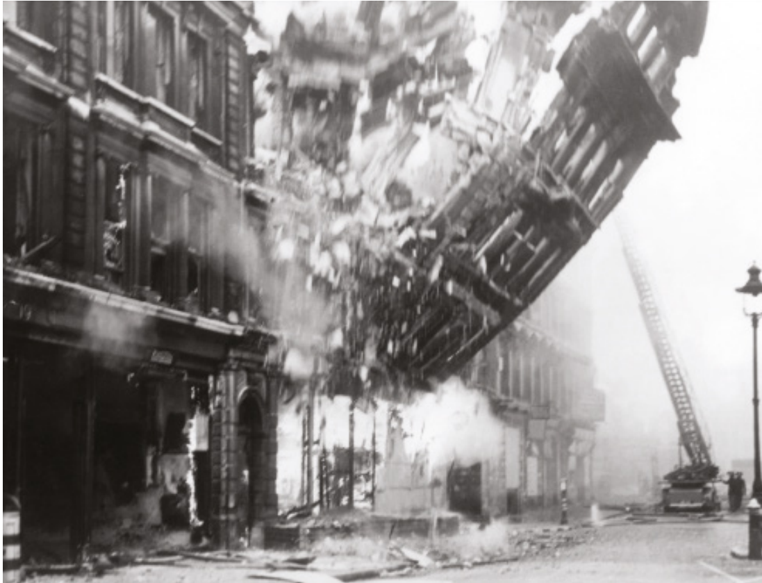
BOMB DAMAGE AT QUEEN VICTORIA STREET, 1941
