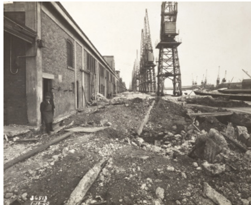
AIR RAID DAMAGE AT ROYAL ALBERT DOCKS, 1940 © PLA collection/Museum of London
