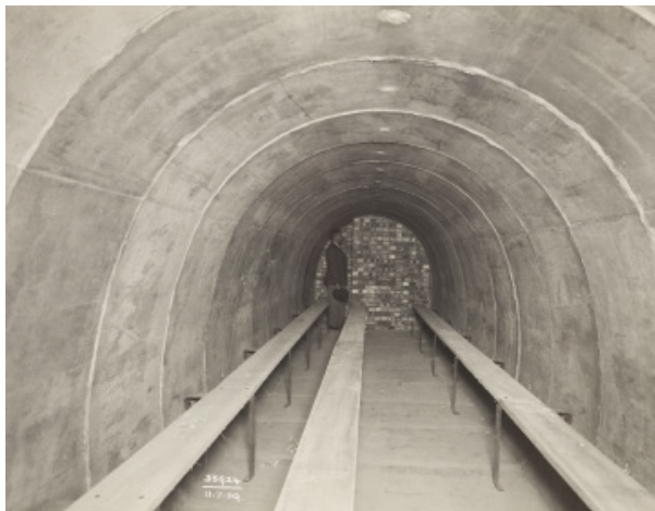
CONCRETE SHELTER AT ROYAL DOCKS
