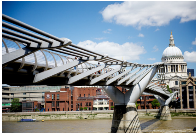
THE MILLENNIUM BRIDGE
