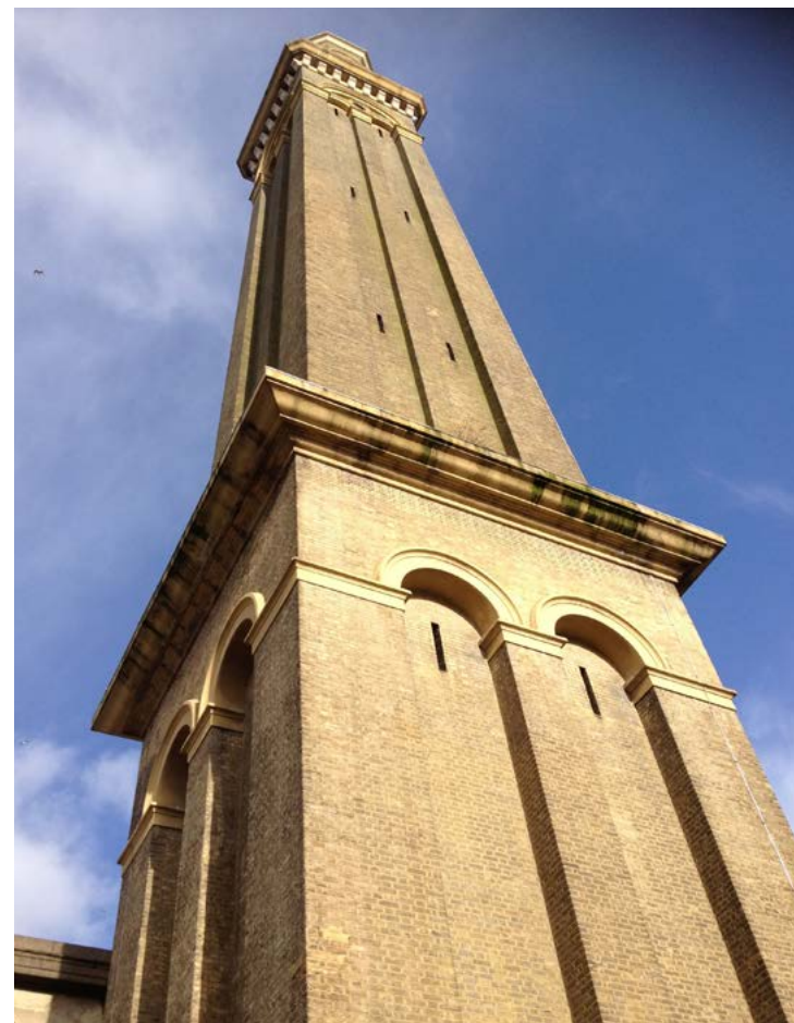
STANDPIPE TOWER AT LONDON MUSEUM OF WATER & STEAM
