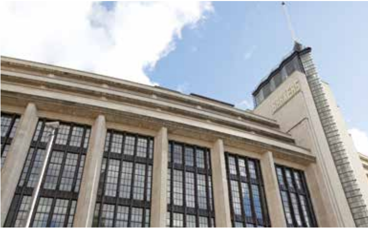
Former Barkers Department Store
