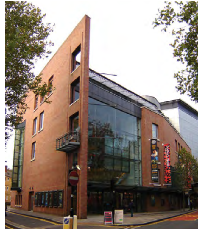
SADLERS WELLS THEATRE Tarquin Binary, Wikipedia Commons
