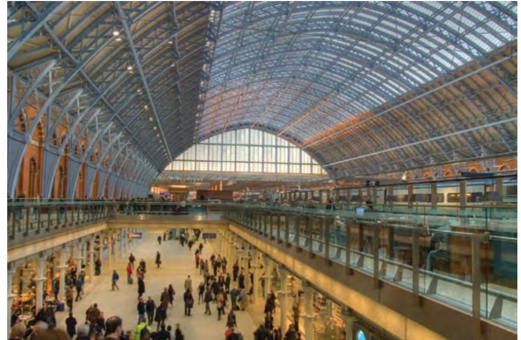
BOMB DAMAGE TO ST PANCRAS STATION. Seanbjack 2007, Flickr
