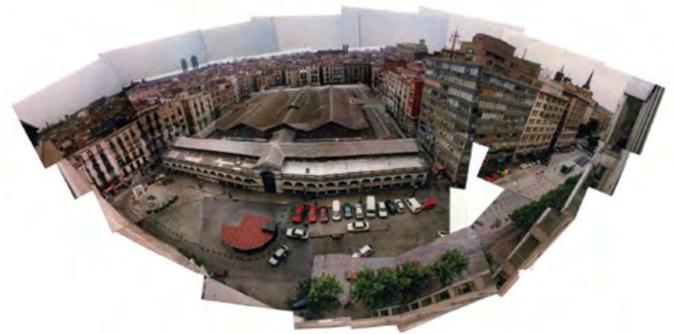
SANTA CATERINA MARKET ROOF BEFORE THE RENOVATION
