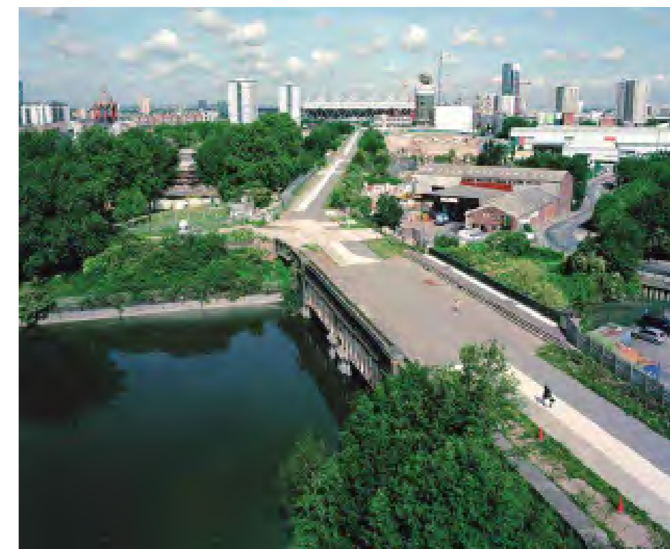
Figure 5.8 Greenway, Stratford providing a linear open space connecting habitats
