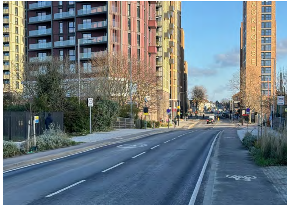
Figure 6.17 Forest Road, Walthamstow comprising street greening, SuDs, cycle lane and footway
