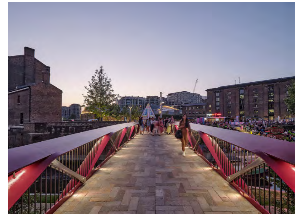
Figure 5.27 Low level lighting that supports person-to-person recognition, Esperance Bridge Kings Cross Image credit Simon Kennedy
