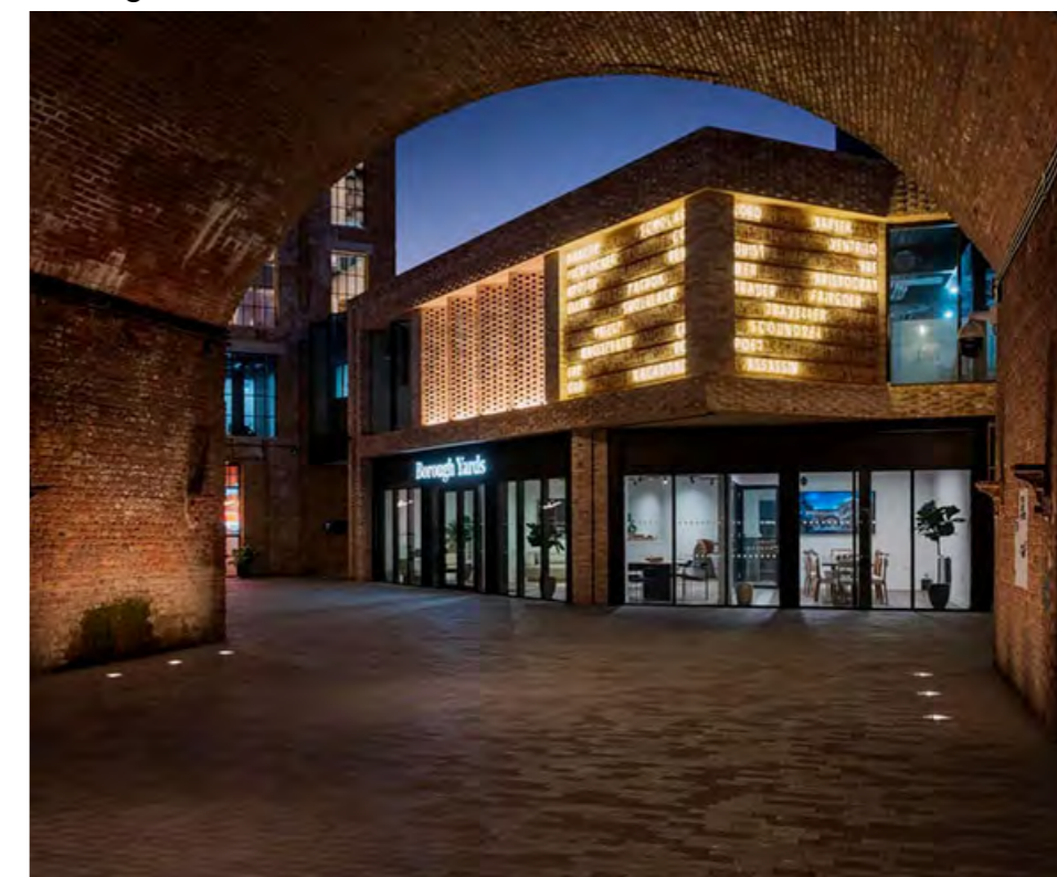
Figure 5.24 Use of materials reflecting local historic character, Borough Yards, Southwark
