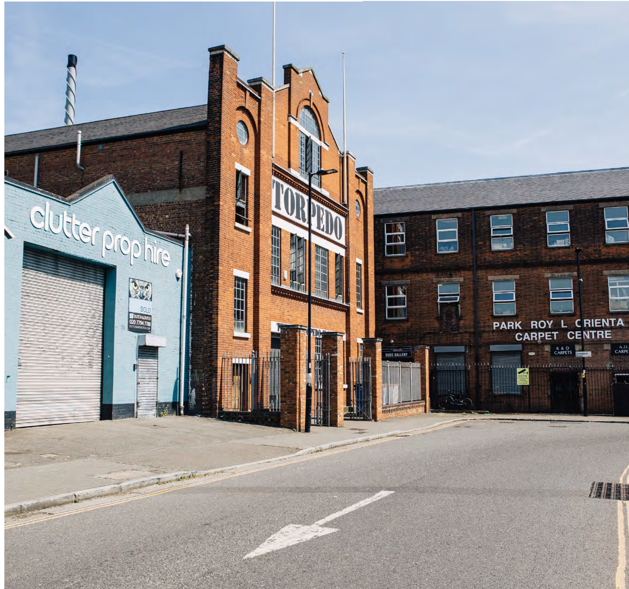
Figure 5.14 Torpedo Factory Locally Listed building in Park Royal
