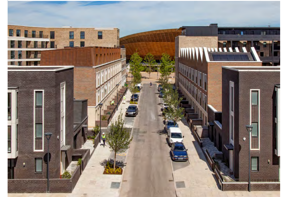
Figure 6.21 Street in Chobham Manor, Stratford exhibiting qualities of a Local Street in a mixed use area
