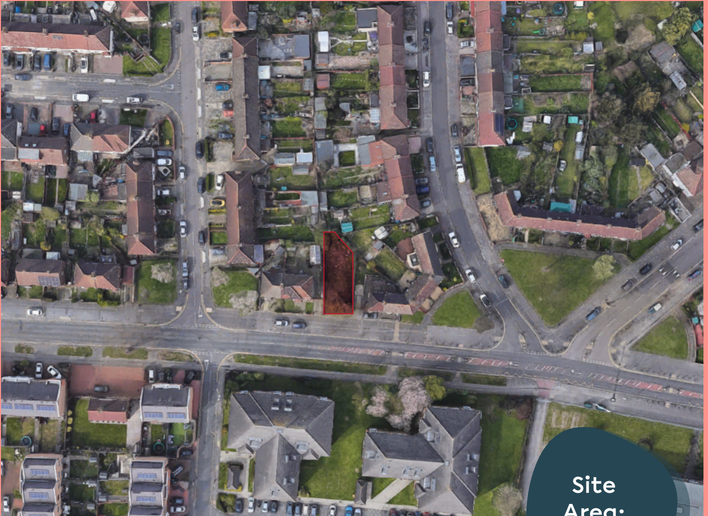
Aerial View over Goresbrook Road site
