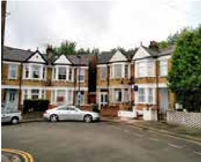
Figure 11.15 Wells House Road
