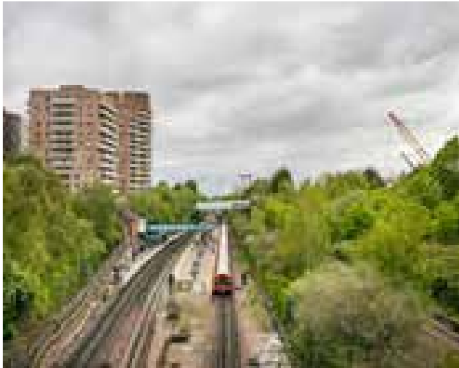
Figure 11.11 North Acton Station
