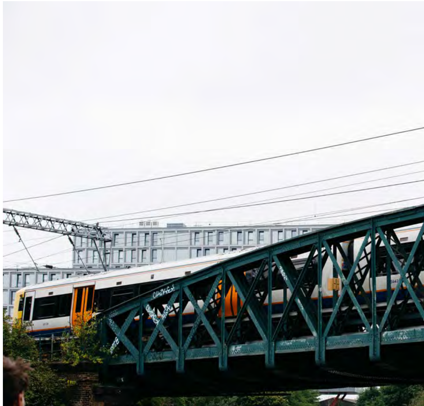
Figure 5.6 Railway bridge crossing the Grand Union Canal
