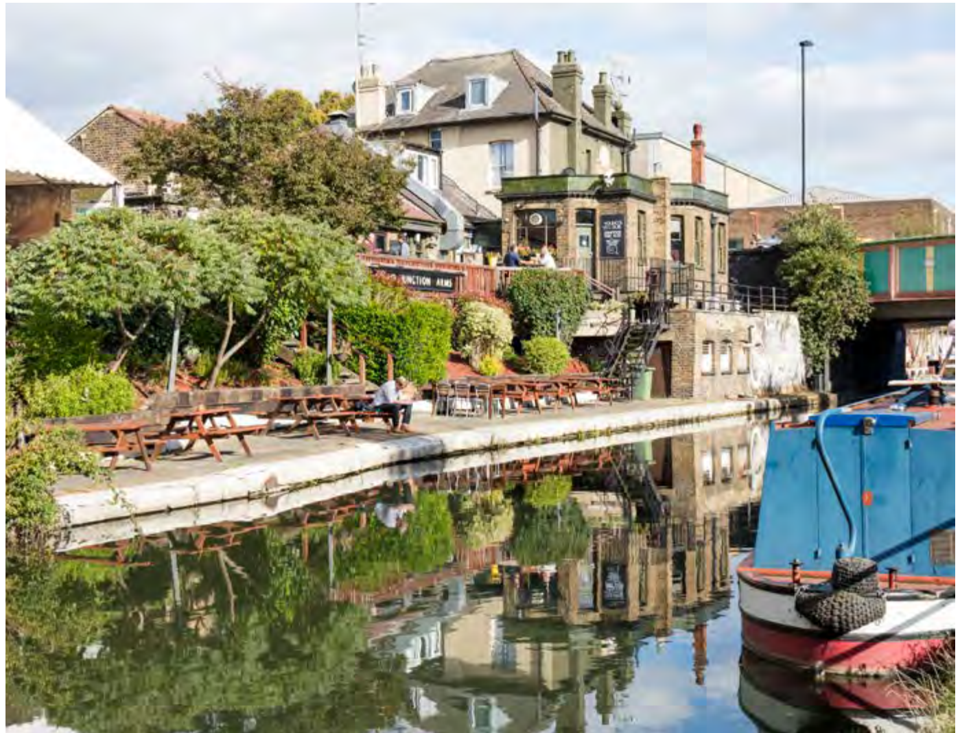
Figure 10.6 Grand Junction Arms providing an existing active frontage to the Grand Union Canal
