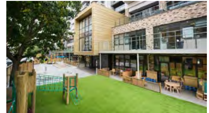
Figure 9.12 Battersea Exchange School
