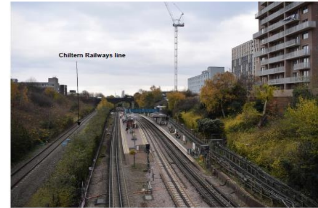
Figure 2.3 View of North Acton Station from Chase Road
