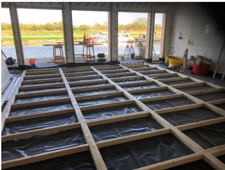
Figure 5: Stokey Energy’s retrofitting work at Leaside Trust
