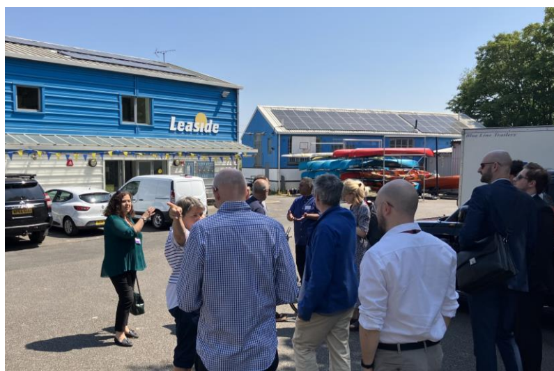
Figure 2: The Leaside Trust, with new solar panels visible on two roofs
