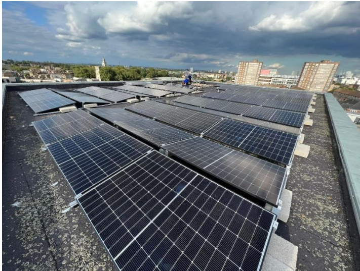
Figure 4: Stokey Energy’s solar panel installation at the Hackney Empire theatre
