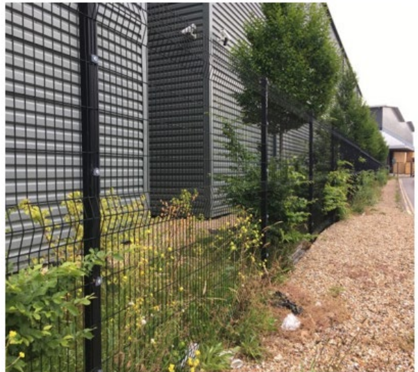
Boundary planting between a new warehouse and an access road.
