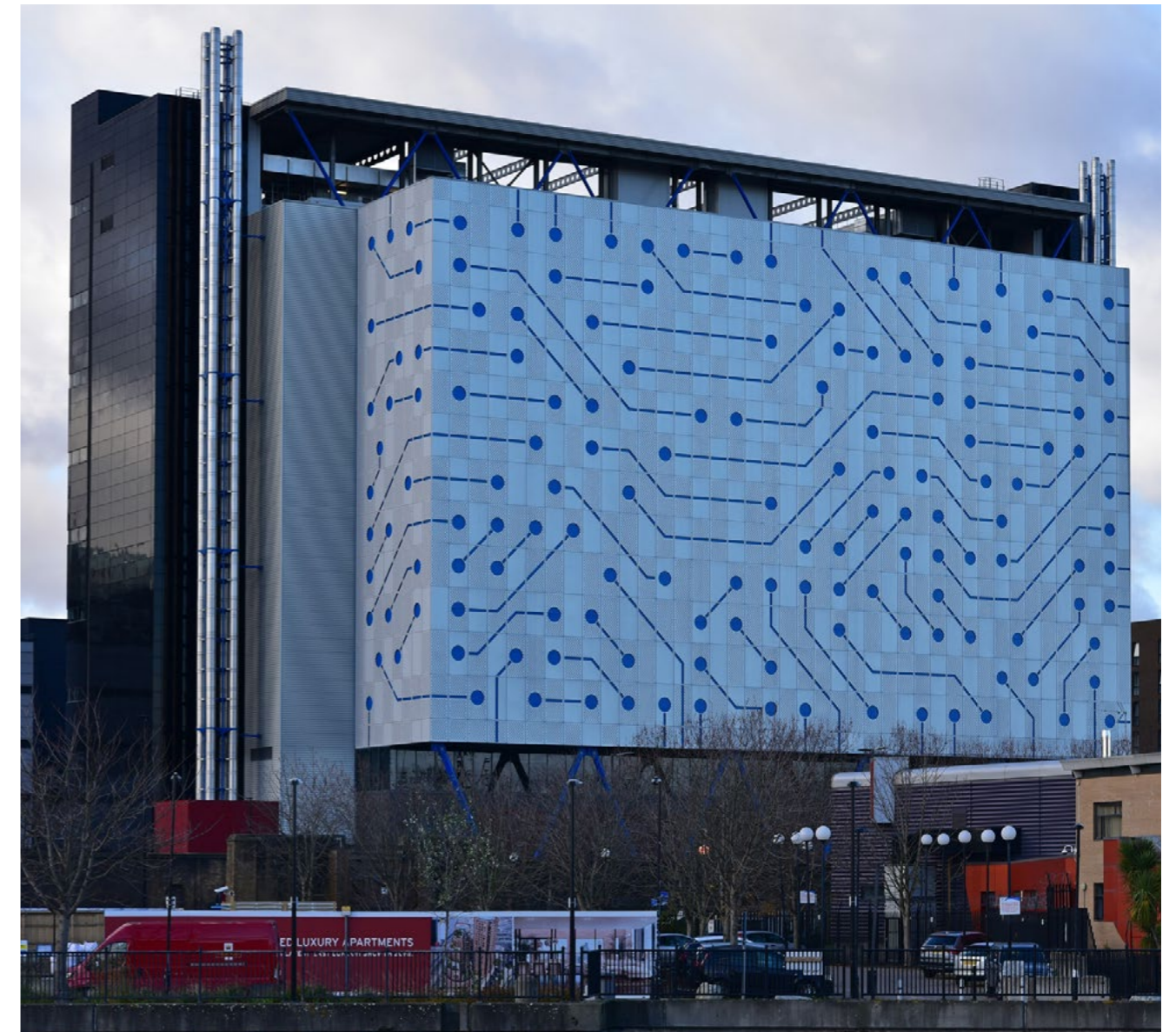
Figure 3.5. Telehouse North 2 Data centre, Tower Hamlets
