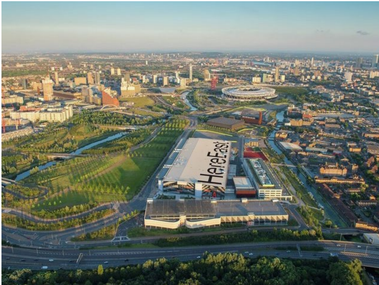
Figure 3.4. HereEast data centre, Queen Elizabeth Olympic Park
