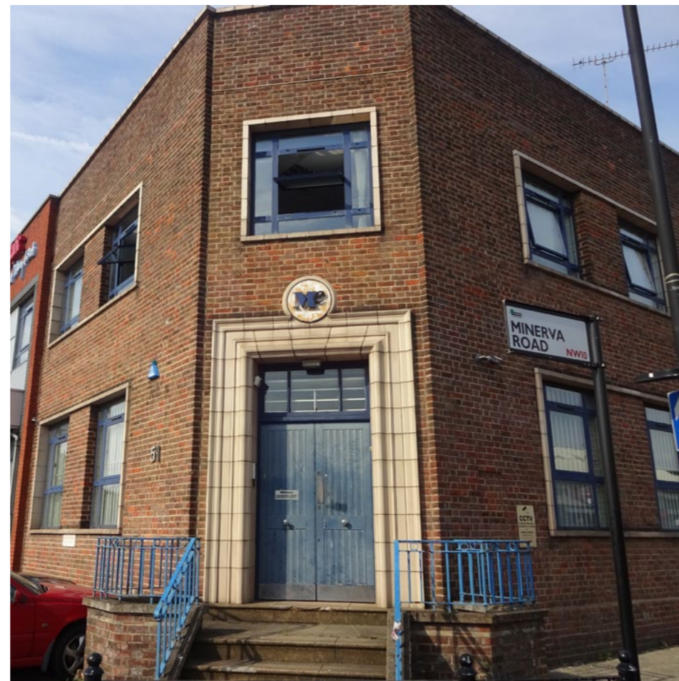
Figure 6.20. Example of a local 1950s industrial frontage
