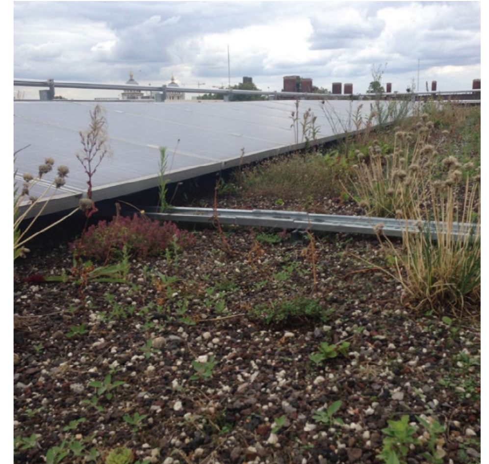
Figure 7.6. Bio-Solar roof providing habitats
