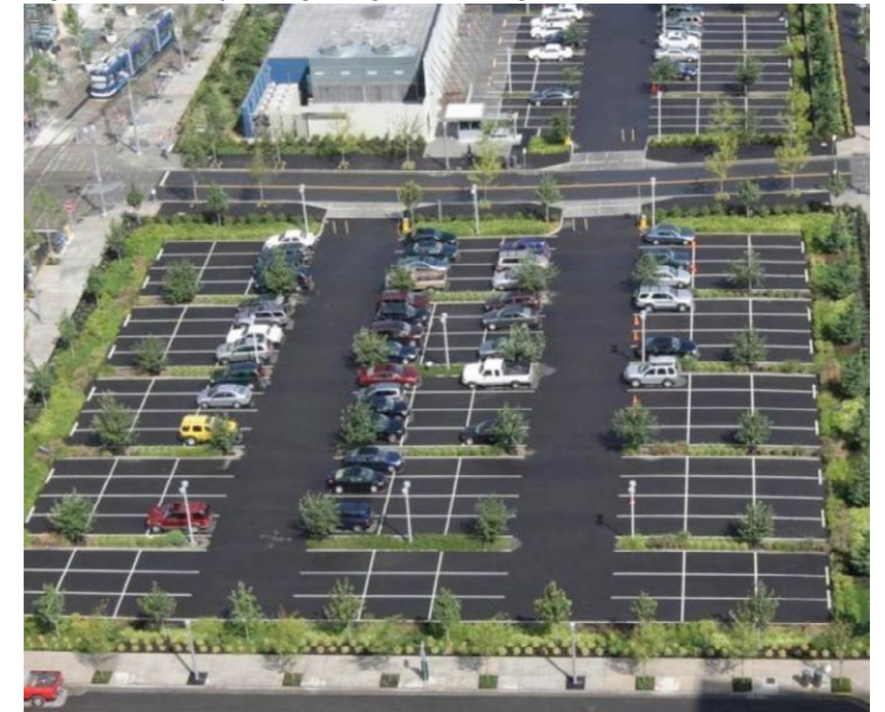
Figure 7.2. Car parking integrated with green infrastructure, USA
