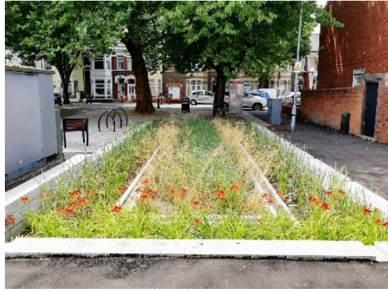
Figure 77: Example of an infiltration basin (Source: Arup).
