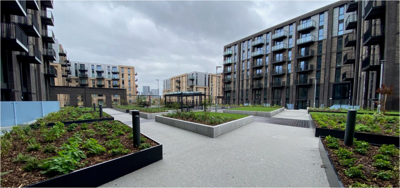
Figure 71: Podium deck blue roof in dense urban development, Middlesdick, Salford (image: abg geosynthetics).
