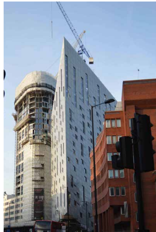
Figure 5.8 Emerging tall buildings at Old Street
