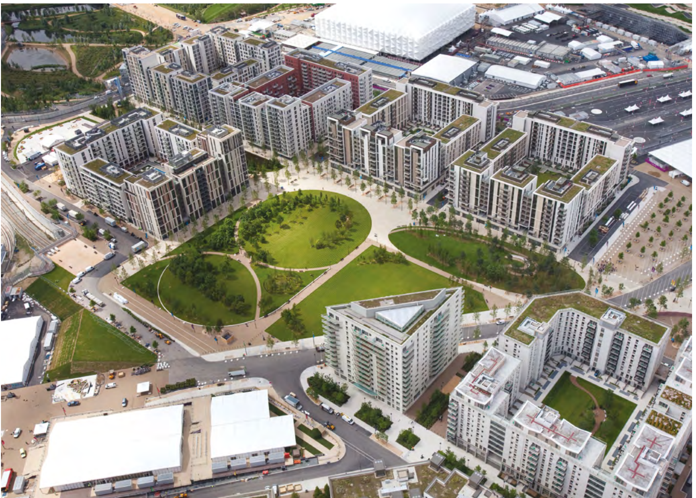
East Village. Managing stormwater and improving water quality through green roofs, bioswales and detention ponds. © LLDC
