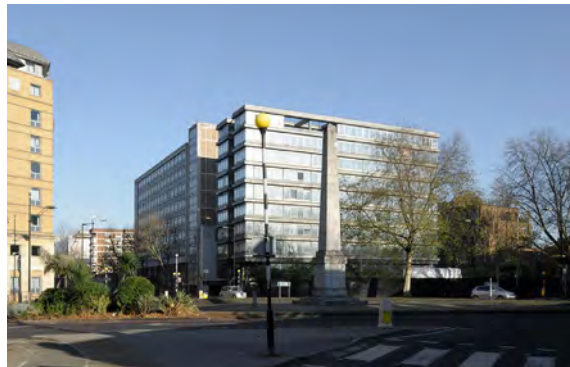
Blackfriars Road, Southwark Existing vacant offices proposed for mixed-use redevelopment
