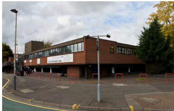
Chiswick Health Centre, Hounslow Existing health centre stacked above a car park
