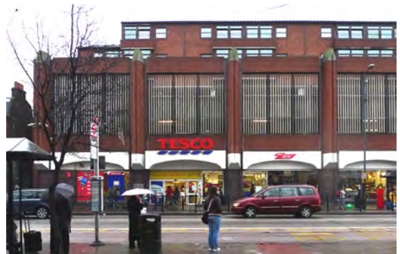
Tottenham High Road, Haringey Residential developed above large-scale retail and car parking
