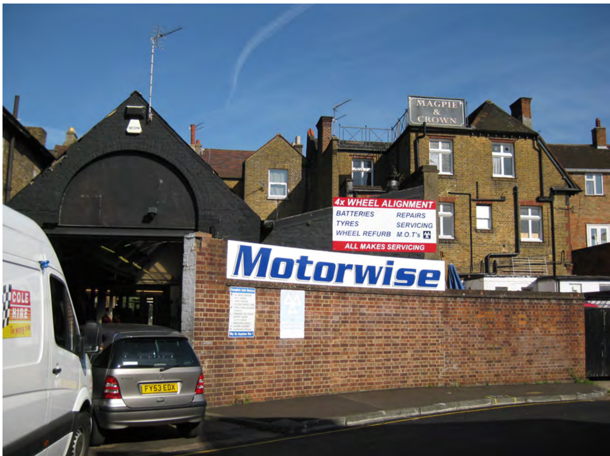
LTES adjoining the rear of Brentford High Street, Hounslow
