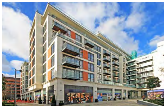
Dickens Yard, Ealing Surface car parking converted to residential
