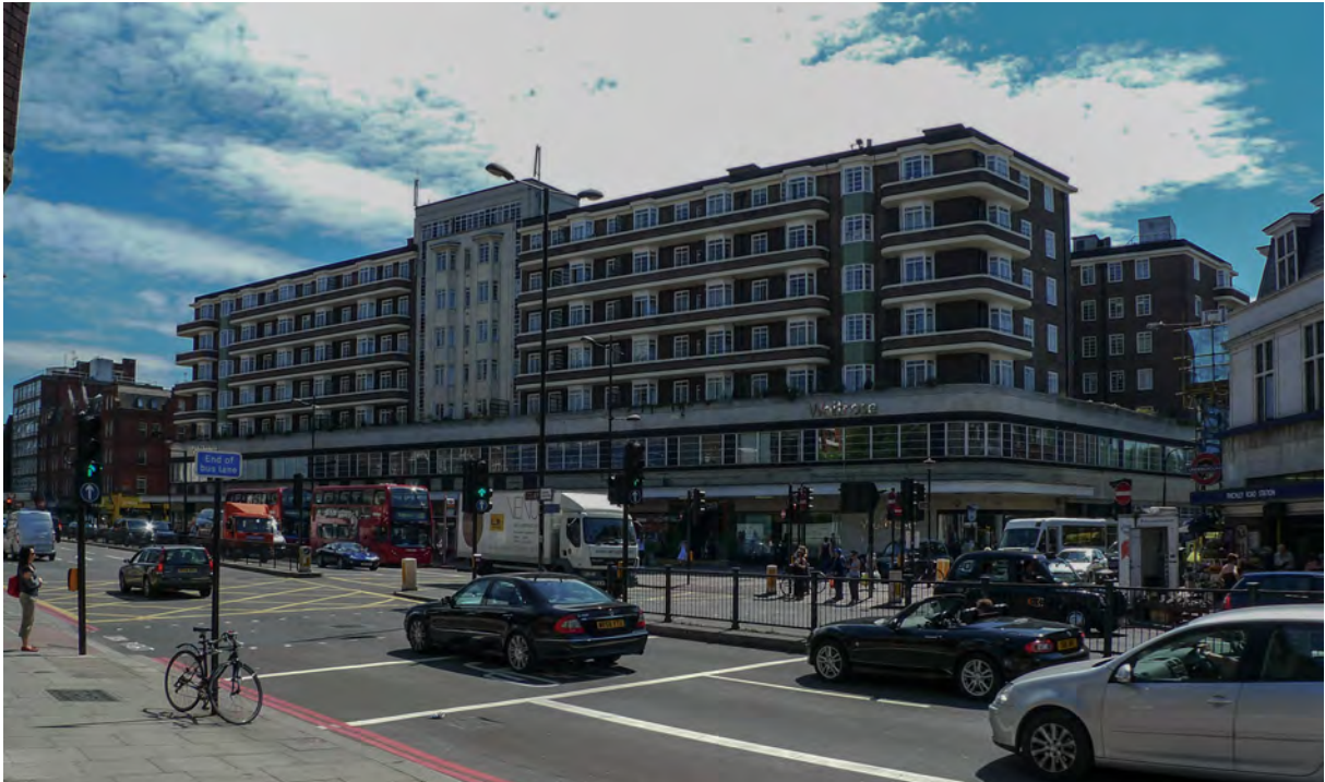
Finchley Road, Camden
