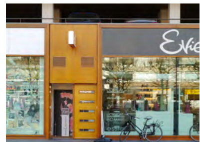
Shops beneath car parking deck
