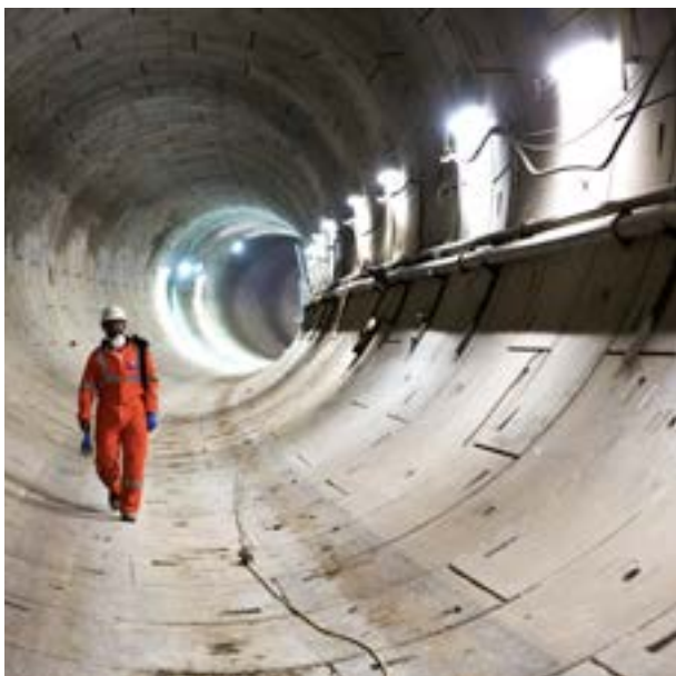
Tunnel inspections near Fisher Street, Holborn. © Crossrail
